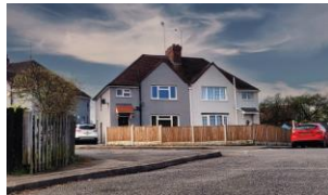
Improving the thermal performance of 92 existing dwellings
