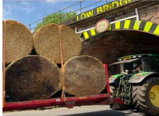
Photo 6 Pinch Point under Railway Bridge
