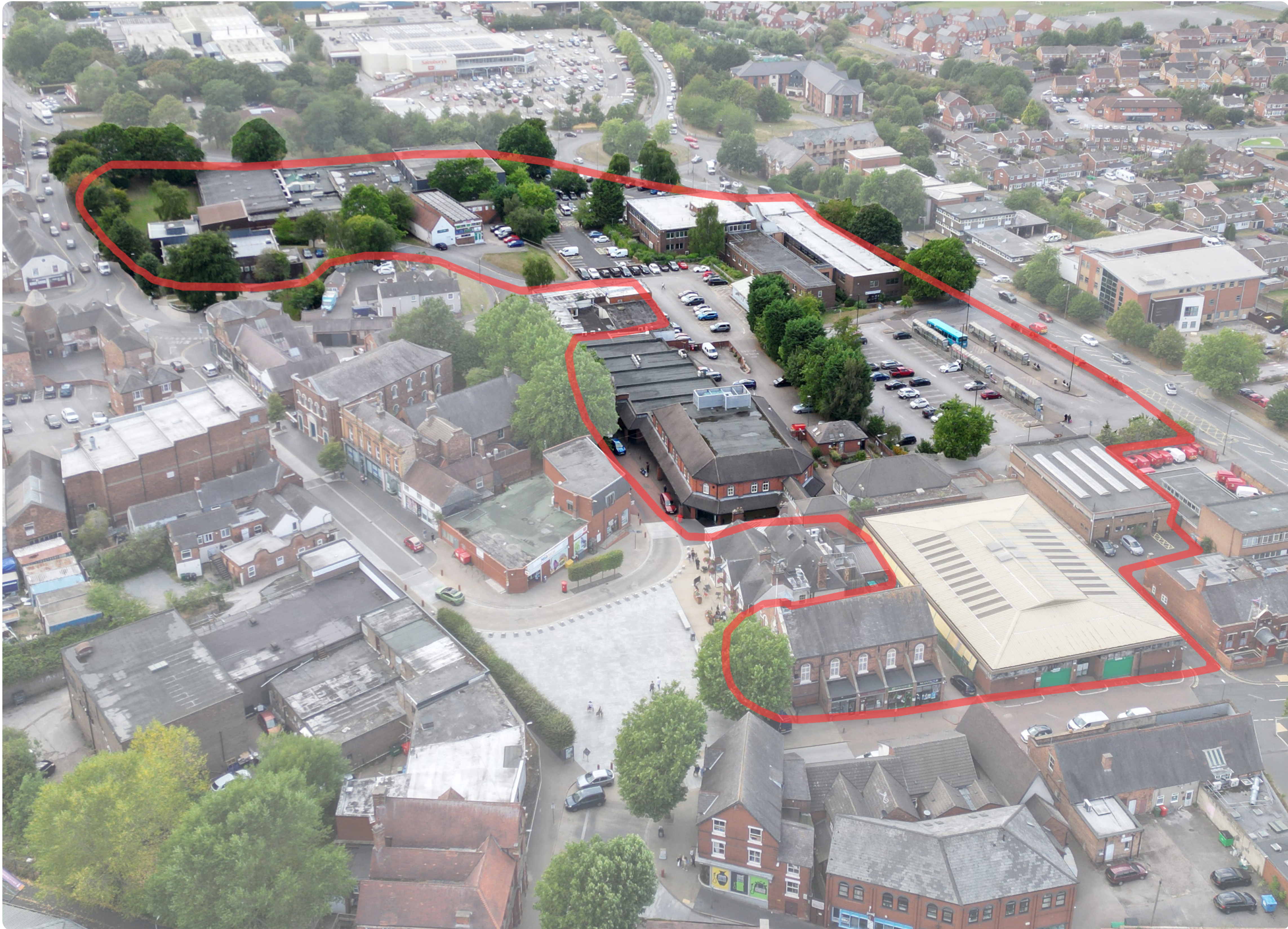
Existing aerial view of the Proposed Civic Site looking from the south-east
