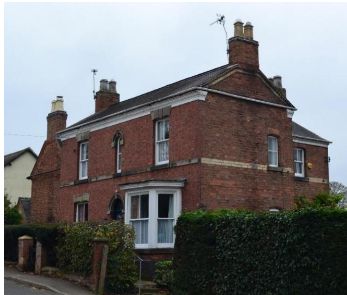
Photo K and L (2): 86-88 Egginton Road, Blakely Cottages
