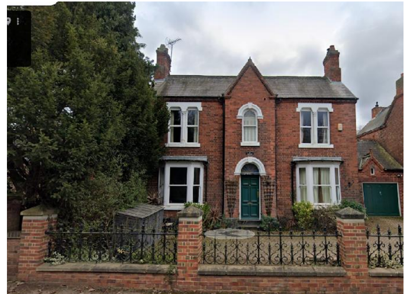
Photo I: 93 Egginton Road (Spring Bank)
