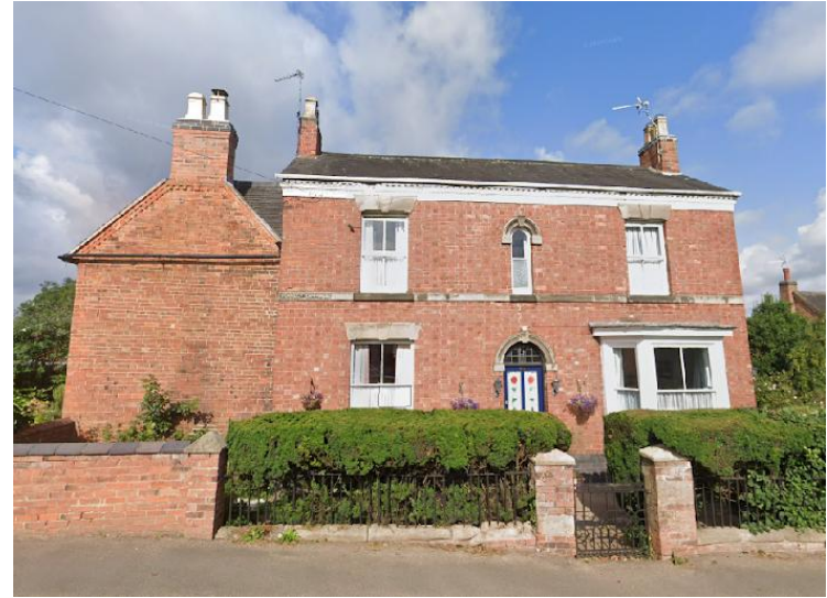
Photo K & L (1): 86-88 Egginton Road, Blakely Cottages
