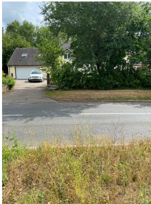
Figure 18 Showing 'Moonraker' A non-designated property to the north of the site.
