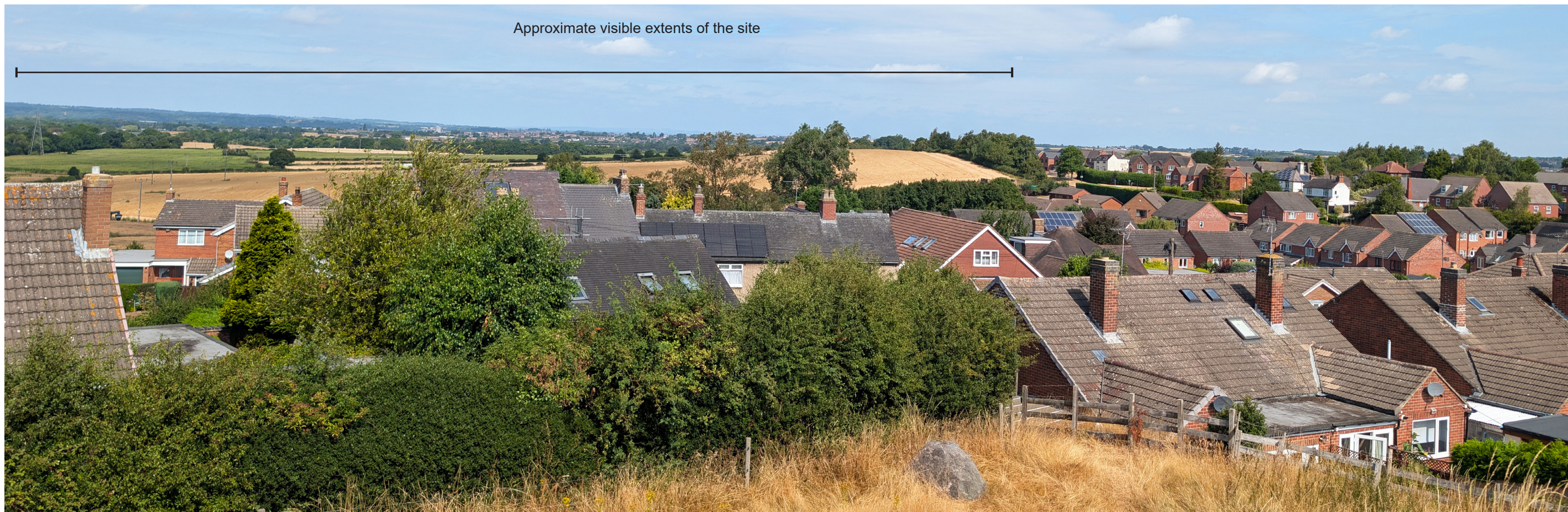
Site 4 View 4: View from Castle Gresley, south-east of the site, looking north-west towards the site.
