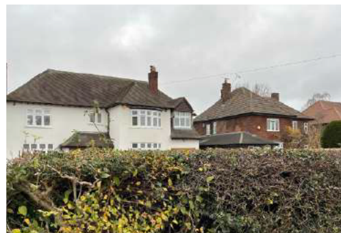
1 Existing set-back detached dwellings fronting Burton Road
