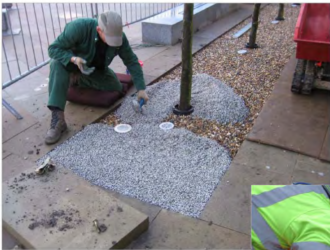
Laying resin bound gravel to tree pits
