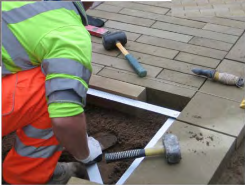
Setting sandstone strips
