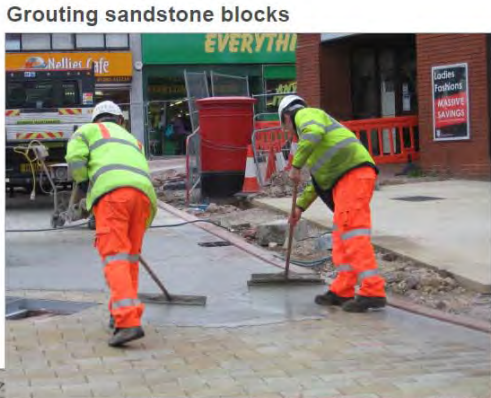
Grouting sandstone blocks
