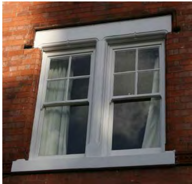
Above - pair of vertically sliding sash windows of 1899 at 1 Shardlow Road. This example incorporates timber horns, which were added to increase the rigidity of the sash frame, particularly when glass panes began to get larger in the second half of the 19th century.
