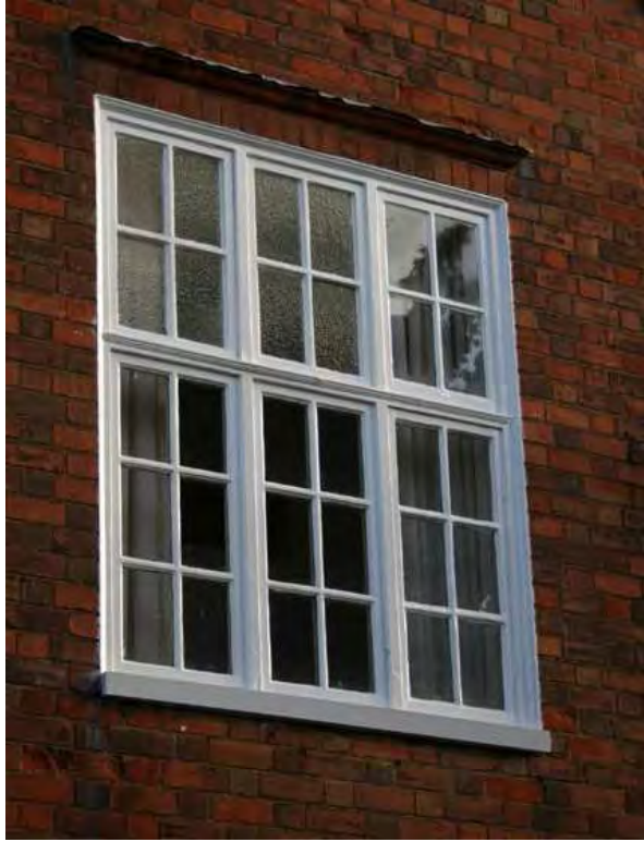
Above - small-paned timber casements within moulded frames (Lodge Mews).
