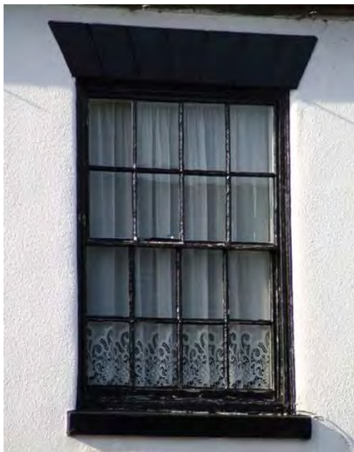
Above - small-paned (8 over 8) vertically sliding sash window at 1 Derby Road.
