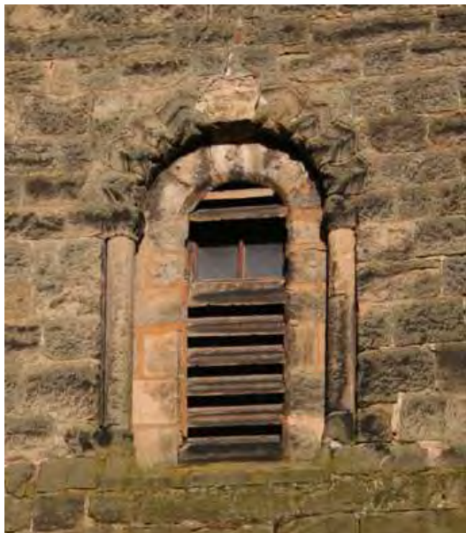
Below left - Norman window opening at the church with chevron mouldings.
