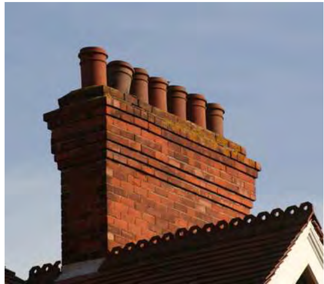
Below left - unusual chamfered brick chimney stack with separate flues and "roll" pots with louvres (25 Derby Road).
