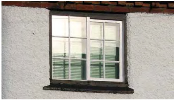
Multi-paned horizontally sliding sash windows, in a number of different patterns. Above - 16 Weston Road. Top right - 2 Weston Road. Below - 34 Weston Road. Right - 21 Weston Road.
