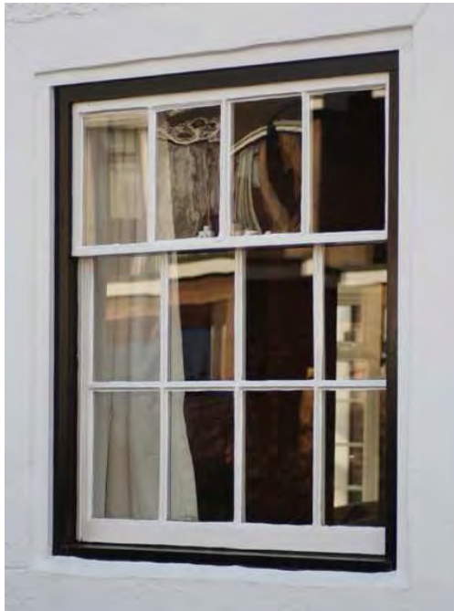
Above - small-paned sash window divided into a third and two thirds (Long Cottage). The lovely reflections of the original cylinder glass are very evident. The same proportions were used at 2 The Green (right).
