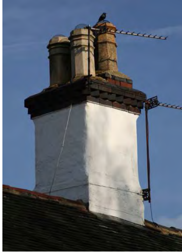
Left - chimney with blue bricks laid in a sawtooth pattern create a decorative corbelled cap. Octagonal buff terracotta pots complete the design (Long Cottage).
