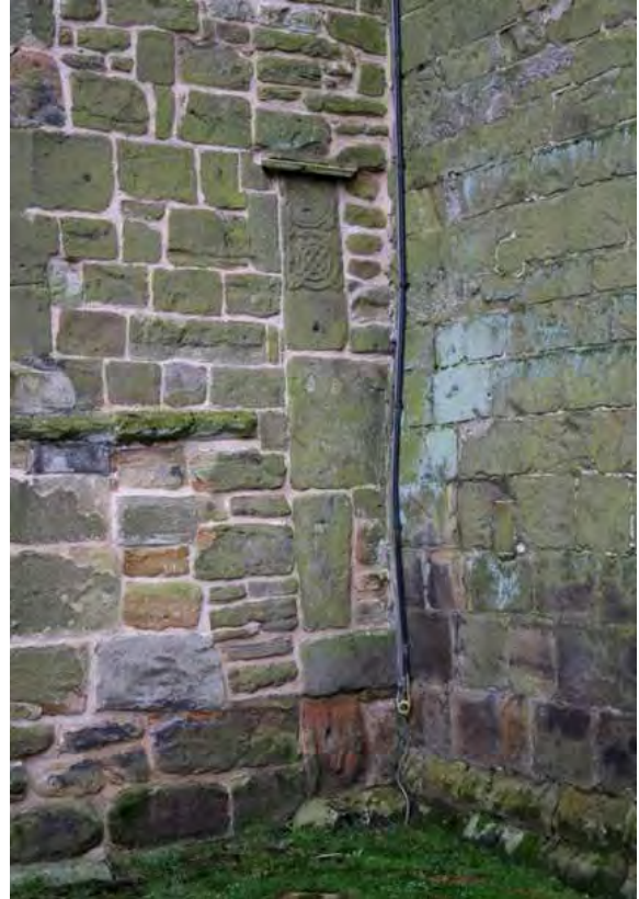
Above right - Saxon stonework incorporating fragments of "long-and-short" work and Saxon interlacing at All Saints Church.
