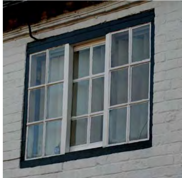
Multi-paned horizontally sliding sash windows, in a number of different patterns. Above - 16 Weston Road. Top right - 2 Weston Road. Below - 34 Weston Road. Right - 21 Weston Road.
