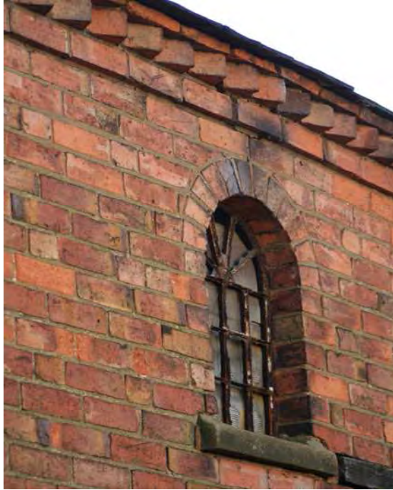
Above - corbelled sawtooth brick eaves and semi-circular arched cast-iron window at 7 Derby Rd.
