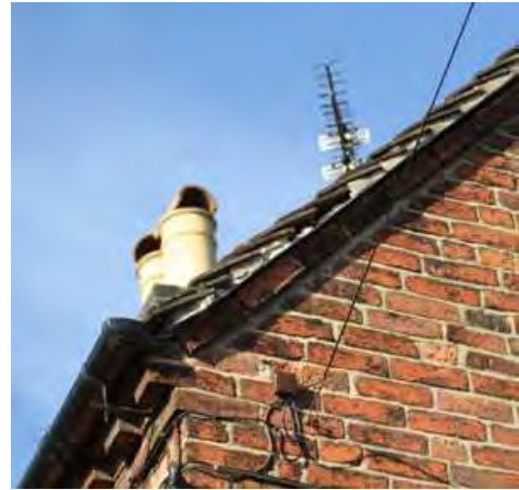
Rounded, moulded brickwork and corbelled verge at The Smithy (top left) and I Manor Farm Mews (above left). Plain corbelled verge (above right) at 28 Weston Rd.
