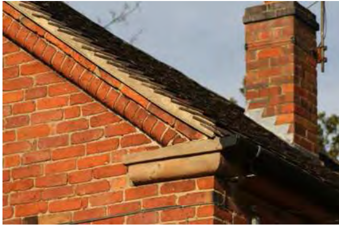
Rounded, moulded brickwork and corbelled verge at The Smithy (top left) and I Manor Farm Mews (above left). Plain corbelled verge (above right) at 28 Weston Rd.
