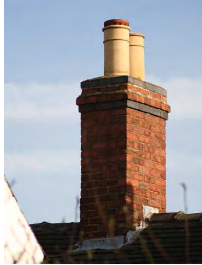
Left - chimney with blue bricks laid in a sawtooth pattern create a decorative corbelled cap. Octagonal buff terracotta pots complete the design (Long Cottage).
