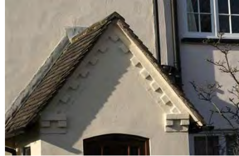
Above - corbelled verge with dentilled brickwork at 29 Derby Road.
