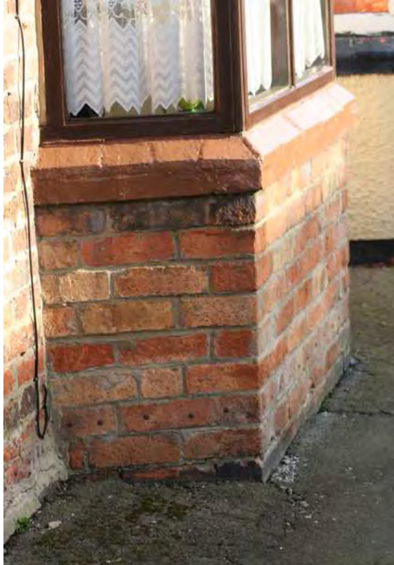
Above left - projecting brick bay with chamfered moulded brick cill, 14 Weston Road.
