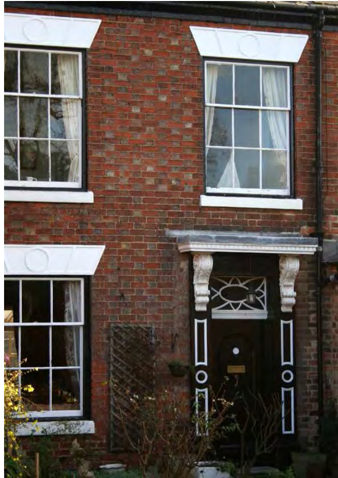
Above - small-paned sash window divided into a third and two thirds (Long Cottage). The lovely reflections of the original cylinder glass are very evident. The same proportions were used at 2 The Green (right).
