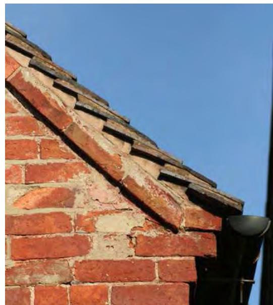
Plain close verge at 20 Weston Road (below left) and corbelled verge at 16 Weston Road (below right).
