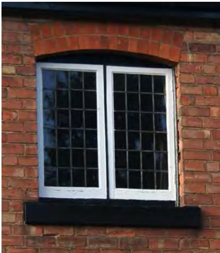
Left - leded-light casement windows in timber frames at 13 The Green. These were re-introduced towards the end of the 19th century as part of the "Arts & Crafts" revival of interest in old building traditions.
