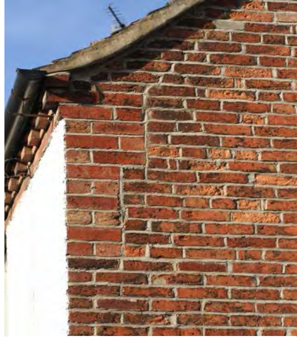
Above right - bricks have been in common use since about 1700. Two phases of brickwork within one wall can be clearly seen at 34 Weston Road (above). It was re-fronted in the 19th century.
