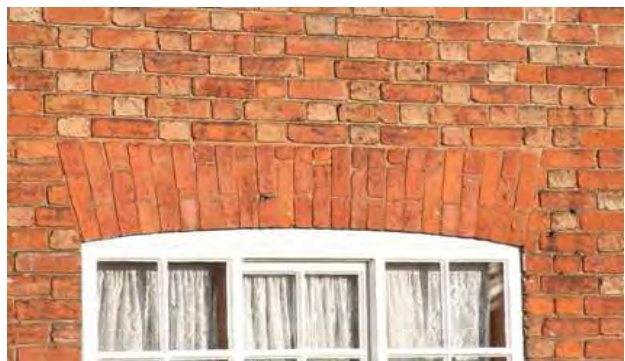
Above - cambered brick arch (2 Weston Road).
