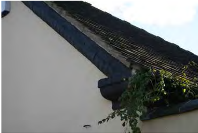
Above - corbelled verge with dentilled brickwork at 29 Derby Road.
