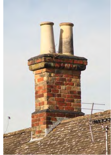
Left - chimney with blue bricks laid in a sawtooth pattern create a decorative corbelled cap. Octagonal buff terracotta pots complete the design (Long Cottage).
