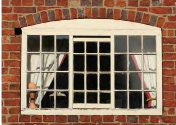
Multi-paned horizontally sliding sash windows, in a number of different patterns. Above - 16 Weston Road. Top right - 2 Weston Road. Below - 34 Weston Road. Right - 21 Weston Road.
