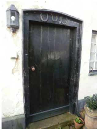
Left - plain Georgian boarded door on Church Lane. Note the heavy frame and broad width of the planks.
