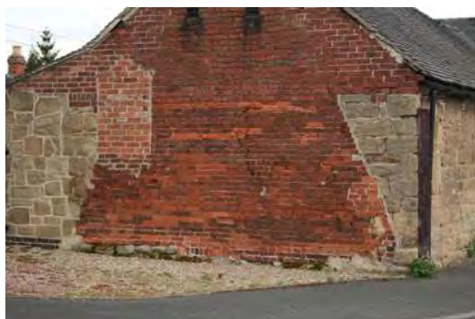
Outbuilding at Walnut Farm
