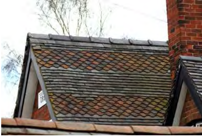
Left - the clay tiled roof at the Old Post Office incorporates bands of plain Staffordshire blue clay tiles alternating with bands of red and blue beaver-tail tiles. This type of pitched roof with bargeboards and these picturesque details were particularly popular during the Victorian period for estate villages.
