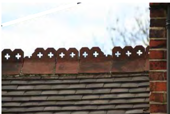
Above left - decorative red clay ridge tiles incorporating a cross pattern (18 Twyford Road). Above right - a gothic, pointed, triangular design (11 The Walnuts). Standardised clay building materials produced in the Potteries and the Derbyshire clayfields became more widely available during the 19th century.
