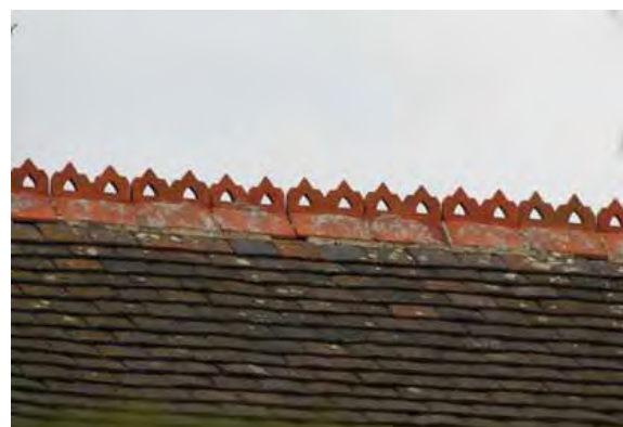
Above left - decorative red clay ridge tiles incorporating a cross pattern (18 Twyford Road). Above right - a gothic, pointed, triangular design (11 The Walnuts). Standardised clay building materials produced in the Potteries and the Derbyshire clayfields became more widely available during the 19th century.
