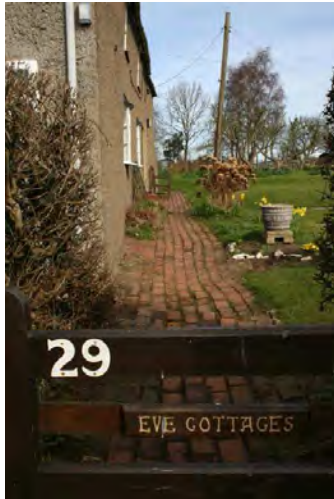
Front wall of Eve Cottages - undulating stone front wall, modern render and red brick path
