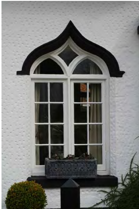
Left - ogee-arched window with timber casements and gothic, chamfered and moulded frame and tracery (Lodge Cottage).
