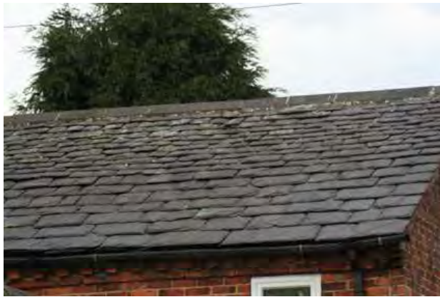
Above left - graduated Westmoreland slate roof at The Pinfold. This material was fashionable for a short period after the Trent and Mersey Canal first opened and may date from the last quarter of the 18th century.
