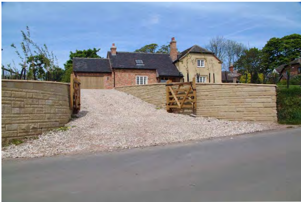
Fern Lea, The Square - stone walls with sharp-edged and snecked courses
