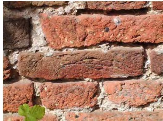
Below - 17th century brickwork from garden wall to Etwall Hall, hand-made in a local clamp kiln.
