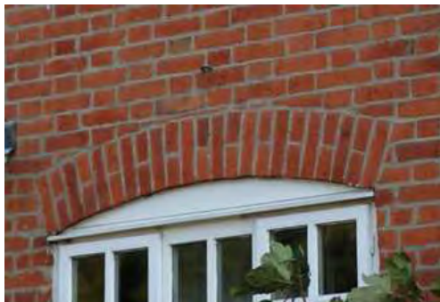
Above - segmental brick arch
