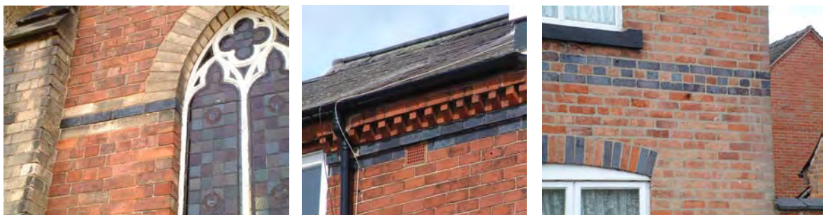
Below - small elements of buff and blue polychromatic brickwork introduced in the late 19th century.
