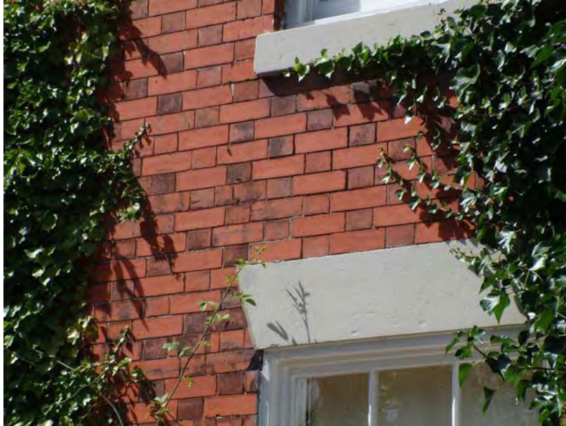
Above - mid 19th century Flemish bond brickwork.
