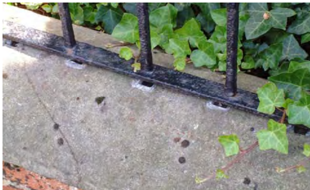
Stone copings (below) and shaped blue brick (bottom).
