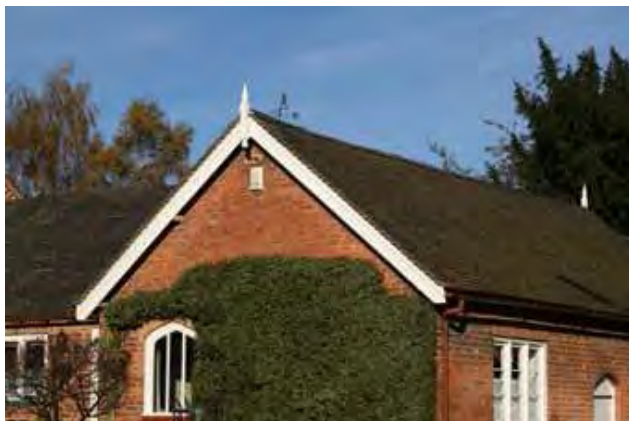
Left - the use of decorative timber bargeboards was commonplace in the 19th century for “picturesque” buildings, such as the former parish room (left), but is rare in Etwall.
