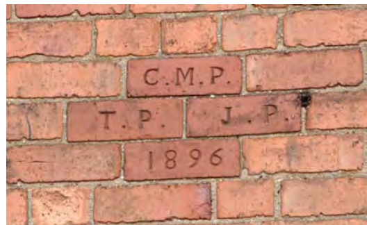
Late 19th century, regular, smooth-faced brickwork with date stamp (above).
