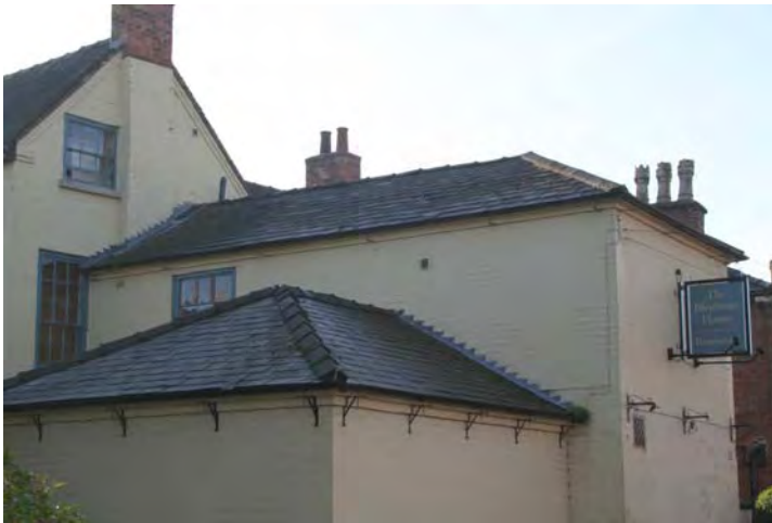
Hipped roofs (left and below) in tile and slate; Main Street, Etwall
