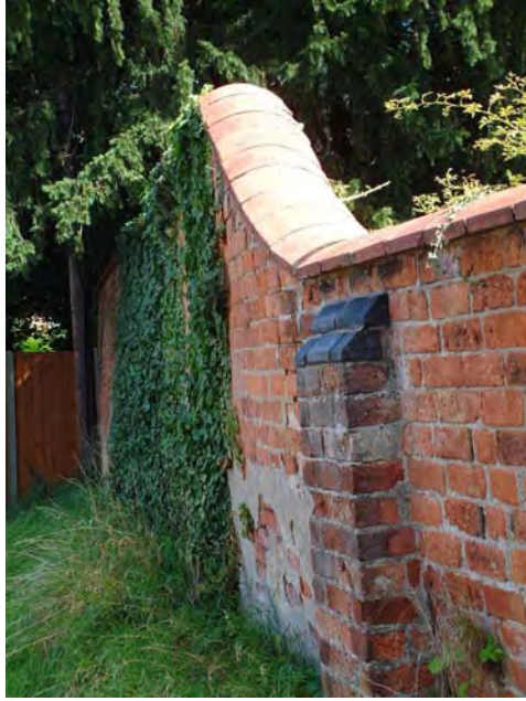
A variety of copings co-exist. Red clay half-round copings (above and middle right) at The Old Rectory.
