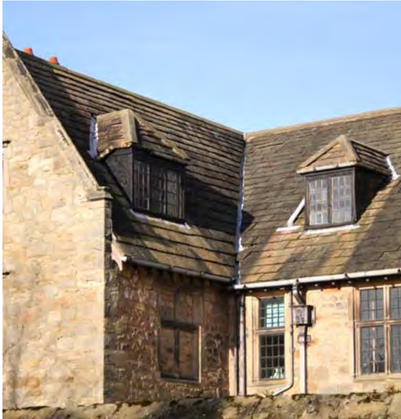
Left - stone slate roof, laid in graduated courses at The Hall. This roof was added to the house when it was rebuilt in the early 20th century. It is the only stone slate roof in the village.
