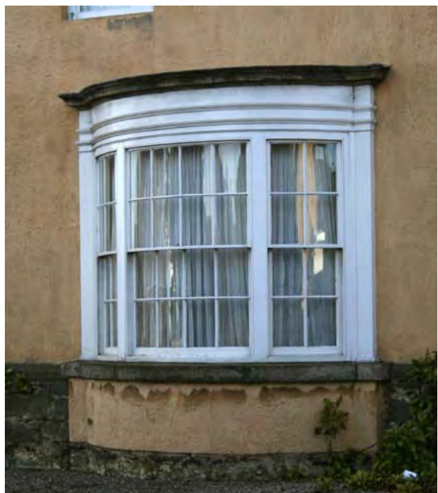
Below - Restored bow window at Kings Newton House, an early 19th century addition, incorporating a tri-partite sash framed by pilasters and moulded entablature.
