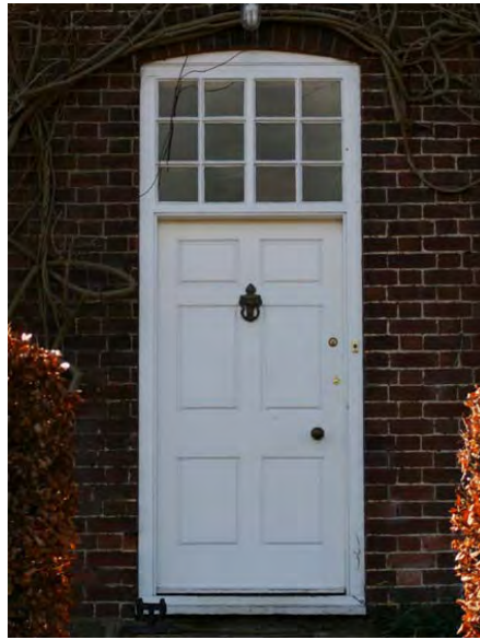
Far left - 18th century boarded door with a panelled frame applied to the face (stableblock at The Hall).
