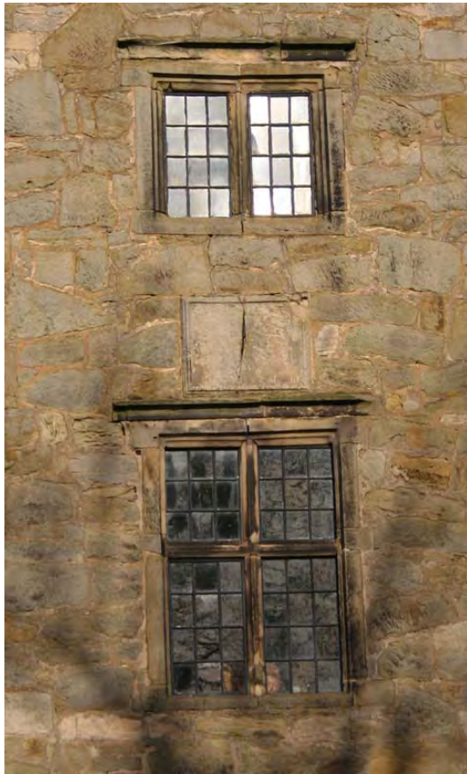
Above - moulded mullioned windows with leaded-light casements at The Hall.
