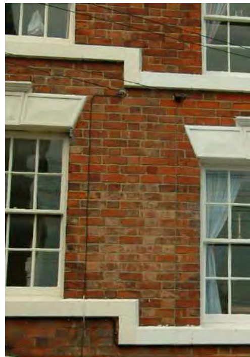
Above - in places, a stone cill was used as a cill band, which runs across a whole elevation or multiple buildings, at 10-18 High Street.
