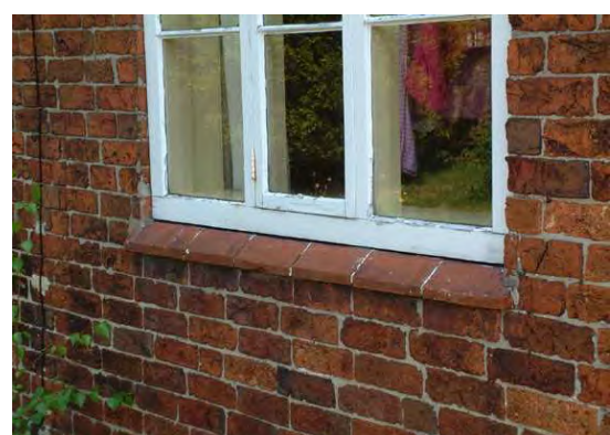
Above - in places, a stone cill was used as a cill band, which runs across a whole elevation or multiple buildings, at 10-18 High Street.
