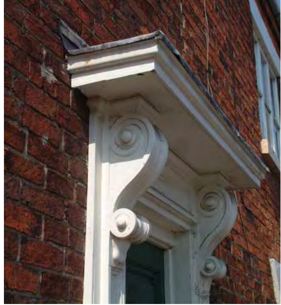
Above - Victorian doorcase, incorporating decorative scrolled console brackets and projecting cornice (49 Derby Road).
