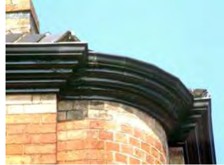
Left - hipped roof with pronounced overhanging timber eaves. Occasionally a more decorative timber eaves was used on the 19th century villas (above).
