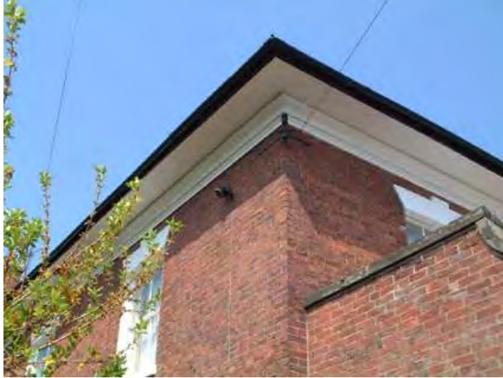
Left - hipped roof with pronounced overhanging timber eaves. Occasionally a more decorative timber eaves was used on the 19th century villas (above).
