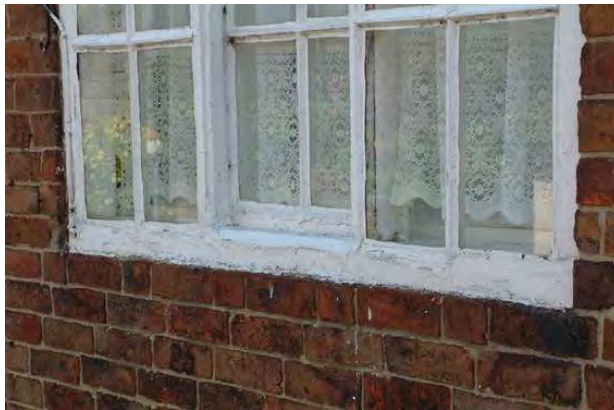
Above - in places, a stone cill was used as a cill band, which runs across a whole elevation or multiple buildings, at 10-18 High Street.
