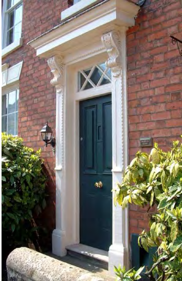
Above - Victorian doorcase, incorporating decorative scrolled console brackets and projecting cornice (49 Derby Road).
