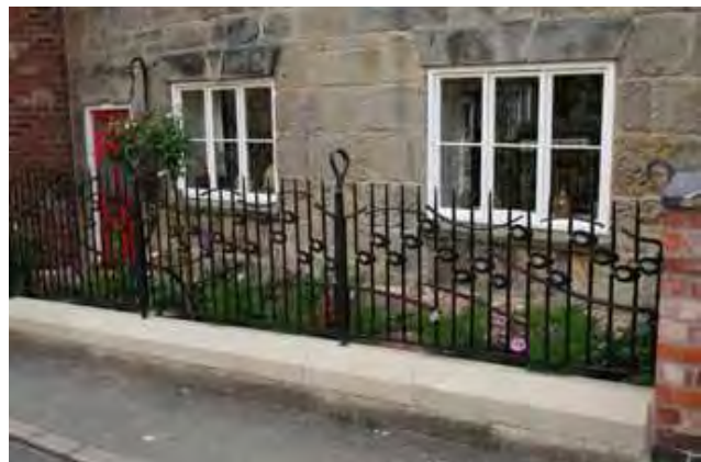
Below right - hand-forged railings in steel; a modern interpretation of wrought ironwork by David Tucker (11 Blanch Croft)
