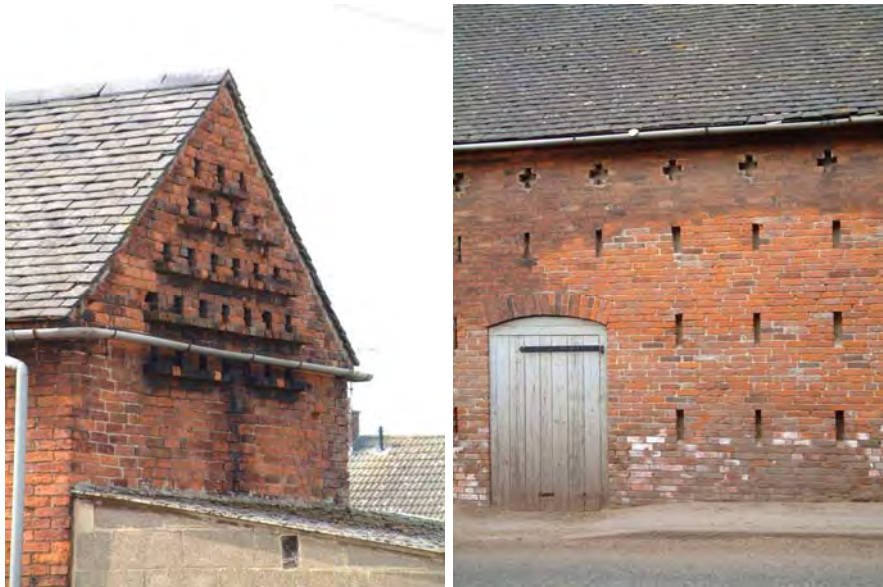
Flight holes for dovecote (left) and ventilation holes in barn (right) at Trent Farm
