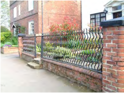
Railings at Mercia, 5 Main Street
