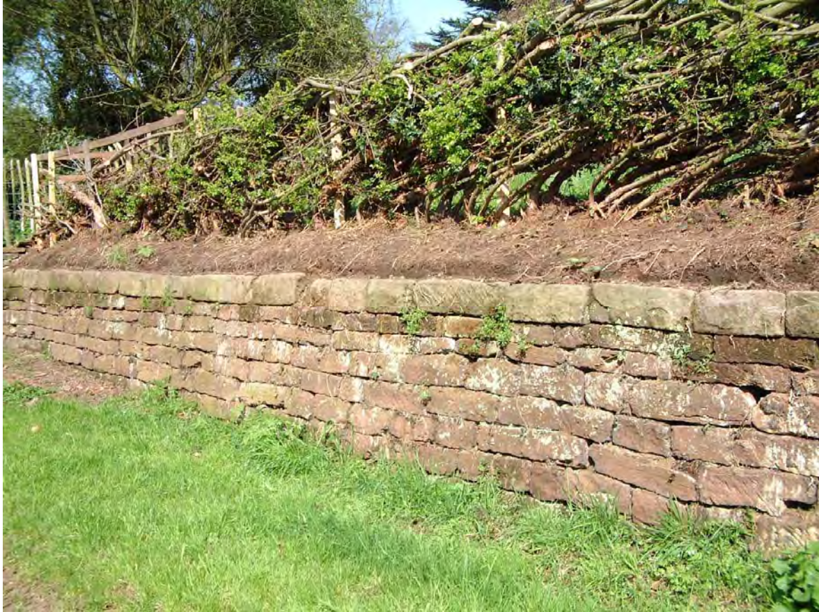
Many of the walls around the Newton Park estate were built in an evenly coursed pinkish sandstone (as at Farm Lane - above).
