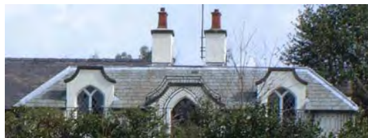
Pitched roofs - verges emphasised with shaped timber bargeboards and finials (above).
