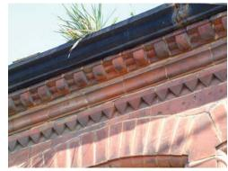
visible brackets as on the south side of High Street. The gutter profile thus became an integral part of the architecture of the building. The detail is very attractive, but lack of attention to leaking joints can cause the brickwork below to become saturated and vulnerable to frost damage. As with the detail last described, some examples have been replaced with half-round uPVC.
