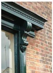
Above, left and right - traditional pilasters. console brackets and cornices. These elements of traditional shopfronts include a plethora of designs with acanthus leaves, triangular cappings to the pilasters, incised trefoils and recessed panels.
