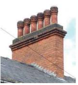
more durable brick was required (top right). Clay pots in both red and buff clay (cannon-type - left, with louvres - right, and square - top).
