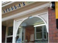
brick stall riser (many over-painted). The abolition of the tax on glass in 1845 was an incentive to use larger sheets of glass. A common detail is the use of timber "spandrels" (curved arched panels) at the top of the window frame which gave the shopfront added strength.
