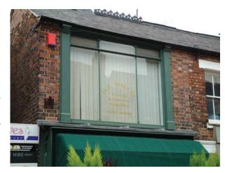
At 8-24 High Street the windows are tripartite sashes, installed to allow as much light as possible into the first floor accommodation. First floor shopfronts have been used at 26, 26a and 55 High Street. These were enabled through the development of internal cast-iron column supports to enable the shopfronts to be treated as curtain walls.
