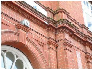
Left - architectural red terracotta incorporating classical elements; entablature, cornice and pilasters, with dentil moulding
