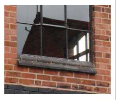
(painted white). Above right - blue clay cill made from moulded bricks. Bottom right - salt-glazed brick cill made with bull-nosed bricks.
