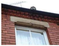
Lintels - moulded stone lintels. In many cases the leading edge of the stone lintel was shaped into a profile incorporating a chamfer or roll-moulding.
