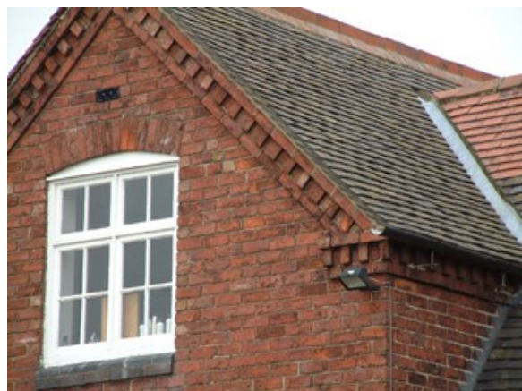
Brick verge details - multiple corbels (above left) corbelled with a single course (above right), corbelled with two courses (bottom left) or corbelled with dentilled brickwork (bottom right)
