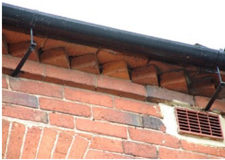
Brick eaves details - dentilled and corbelled eaves (top left), sawtooth and corbelled eaves (bottom left)
