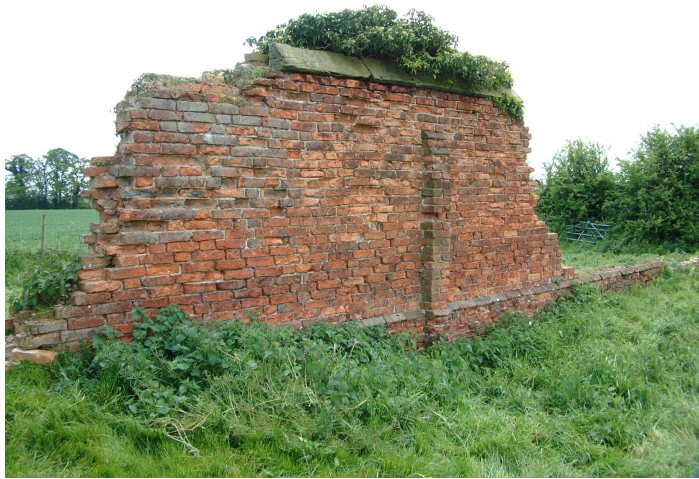
Brick boundary walls (left). These walls, built from long, thin bricks, with an ashlar coping, are fragments of the probable early 17th century kennels and kitchen garden at the former Swarkestone Old Hall.
