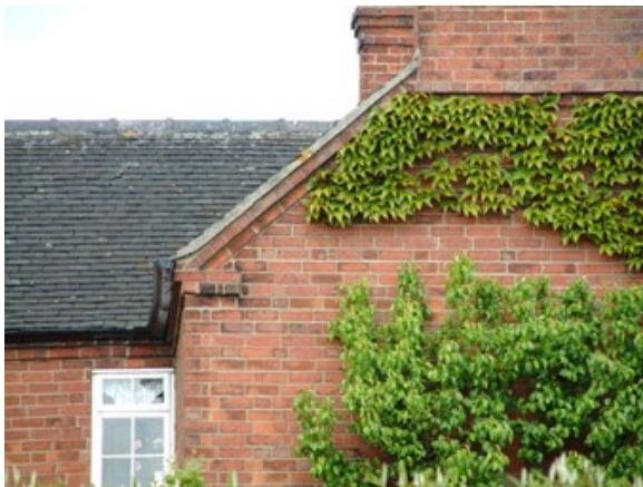
Brick verge details - multiple corbels (above left) corbelled with a single course (above right), corbelled with two courses (bottom left) or corbelled with dentilled brickwork (bottom right)
