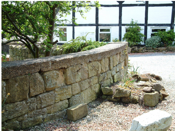
Concrete copings, Woodshop Lane
