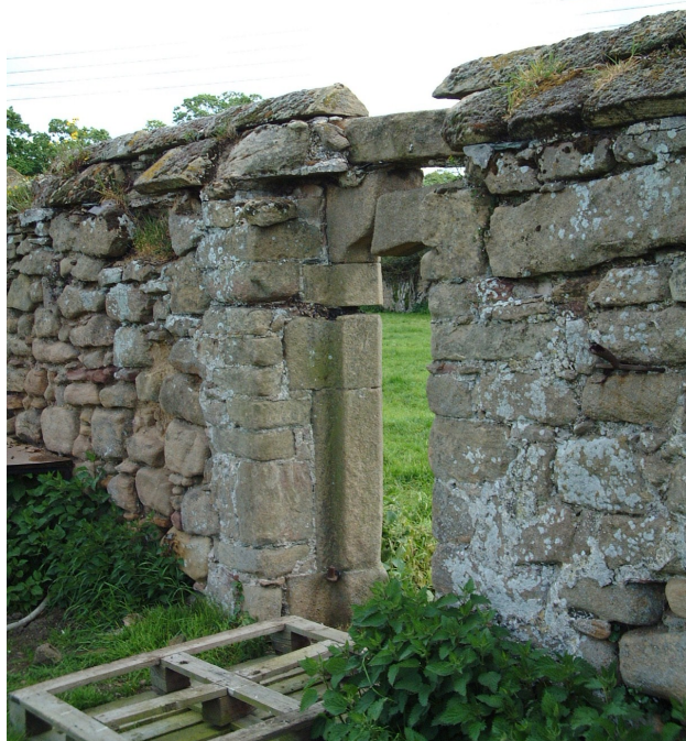
Stone walls to former gardens at the Old Hall (right). Mortared walls built of large blocks of sandstone with copings laid in two courses, of triangular section with a weathering. Shallow arched lintel over doorway with rebated stone jambs may have once been an internal door.
