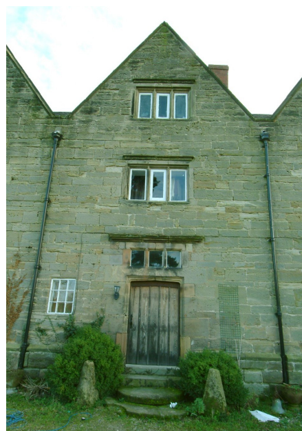
Steep roof pitches at Old Hall Farm
