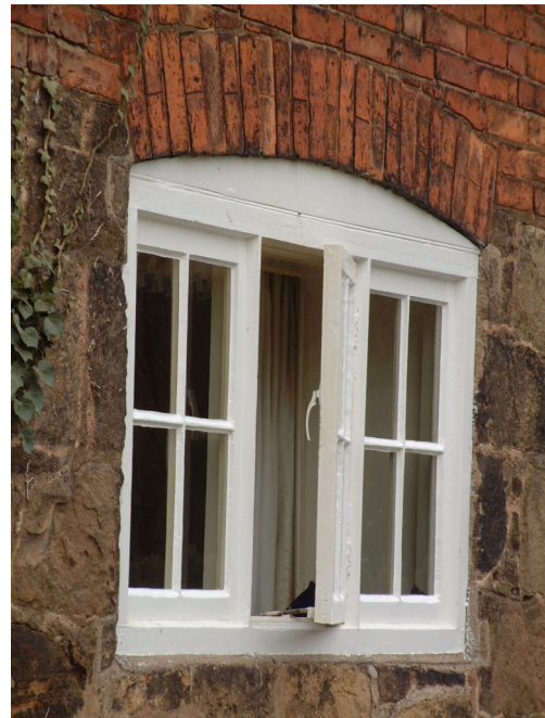
Harpur Crewe estate casement window with chamfered frames
