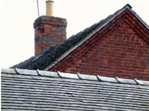
Brick verge details - multiple corbels (above left) corbelled with a single course (above right), corbelled with two courses (bottom left) or corbelled with dentilled brickwork (bottom right)
