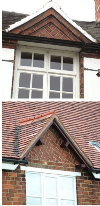
Brick eaves details - dentilled and corbelled eaves (top left), sawtooth and corbelled eaves (bottom left)
