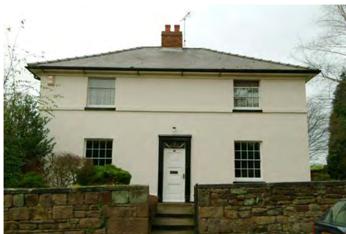
The Firs, High Street: Hipped slate roof and broad overhanging eaves
