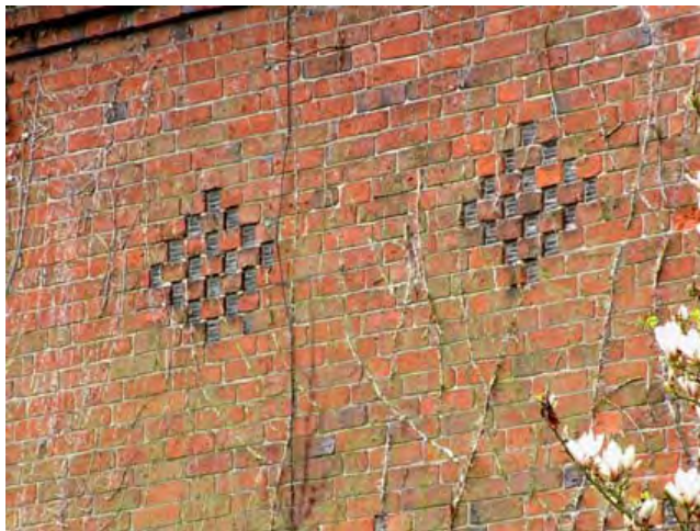
Above - barns often incorporate “breathers” - gaps in the walls to provide cross ventilation. These are often treated decoratively, such as the diaper pattern above. Most examples have been blocked up (as above) with a contrasting material.
