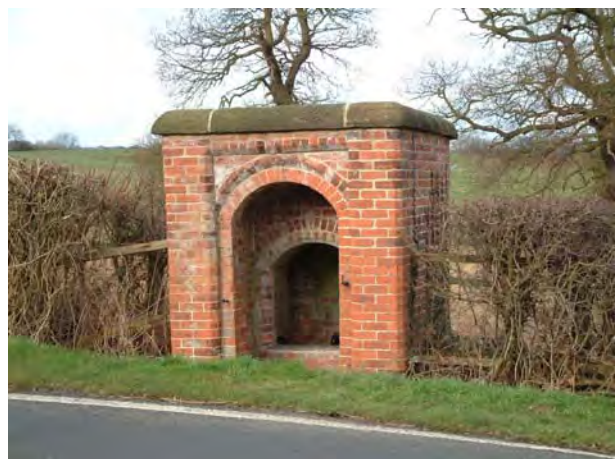
Below left: Remains of well, built in brick and contained within wall of paddock, probably designed to protect a cast iron tap (removed) Below right: Brick alcove containing spring-fed well, early-mid 19th century.
