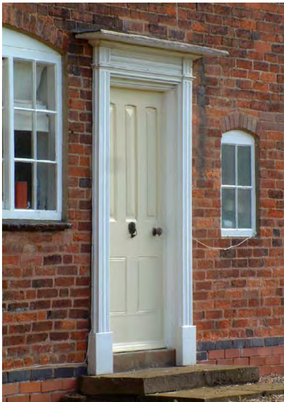
Below left - five-panel Victorian door, the bottom two pales have “scratch” mouldings, whilst the upper panels have “chamfer-stop” mouldings and “raised and fielded” panels. Slender pilastered timber doorcase with mouldings. Below right - gothic style boarded door at 10 Church Lane, with pointed arched top rail, one of only a handful surviving that were adopted by the estate.
