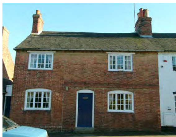
41 High Street - traces of limewash can still be seen under the gutters
