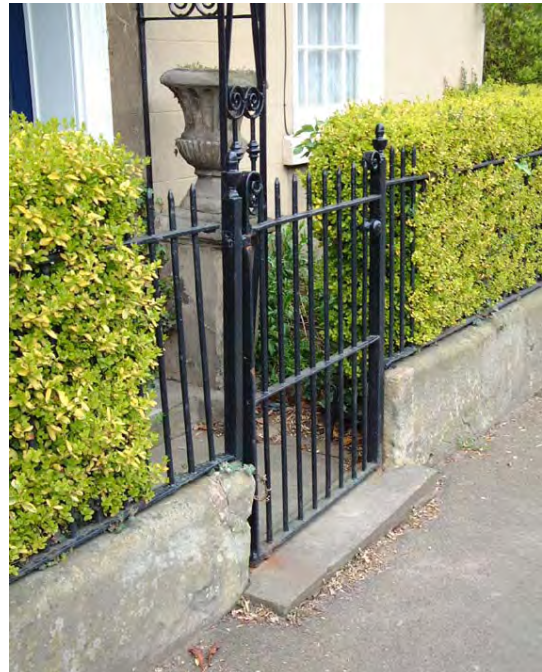
Above and right - iron round bar railings with cast iron urn finials partially concealed by a privet hedge at Pennwyche, 32 High Street.
