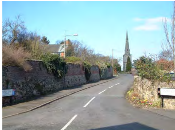
View of the Church from the bottom of Church Lane
