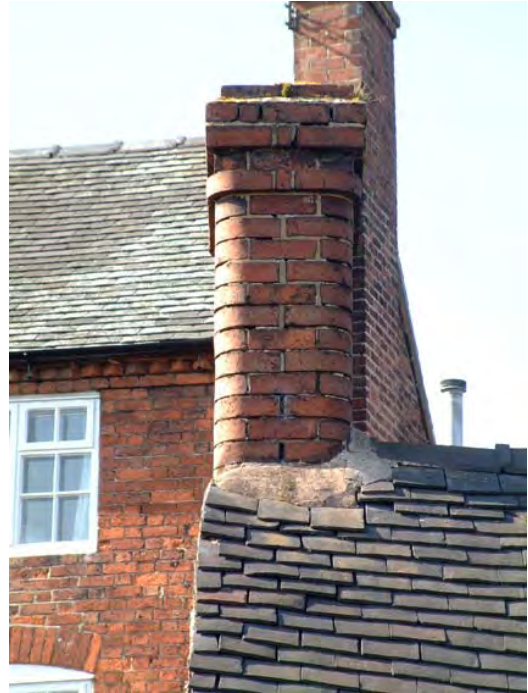
Above and left - a number of buildings and features, such as chimney stacks, were built by the estate with rounded, moulded bricks. These were handmade in special moulds.
