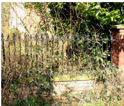
Right - in some instances wrought iron railings were combined with cast iron finials, which could be ordered by the local blacksmith from a catalogue. Here fleur-de-lys finials are combined
