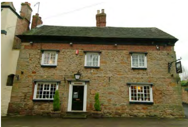
The Chequers Inn built from rubble sandstone and rubble limestone and later raised in brick
