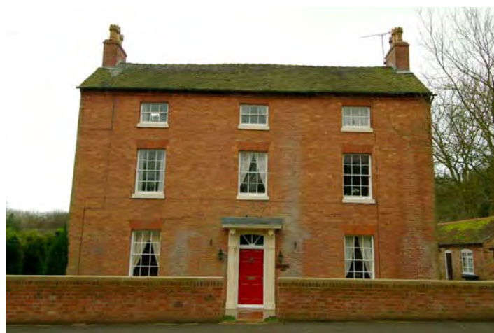
Left - Pennfold Cottage, 8 High Street: Simple segmental arches to ground floor windows, timber lintels at first floor, no cills Right - 124 Main Street: gauged brick arches and stone cills
