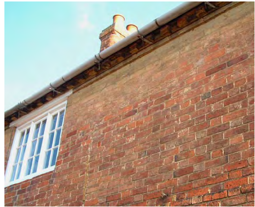
Above and left - a number of buildings and features, such as chimney stacks, were built by the estate with rounded, moulded bricks. These were handmade in special moulds.
