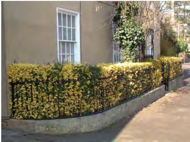
Above and right - iron round bar railings with cast iron urn finials partially concealed by a privet hedge at Pennwyche, 32 High Street.
