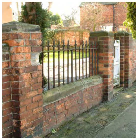
with square section wrought iron railings set straight into a stone plinth.
