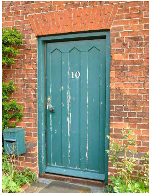
Below left - five-panel Victorian door, the bottom two pales have “scratch” mouldings, whilst the upper panels have “chamfer-stop” mouldings and “raised and fielded” panels. Slender pilastered timber doorcase with mouldings. Below right - gothic style boarded door at 10 Church Lane, with pointed arched top rail, one of only a handful surviving that were adopted by the estate.
