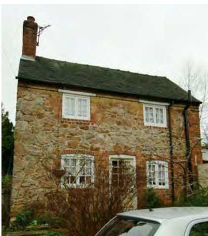
Left - Pennfold Cottage, 8 High Street: Simple segmental arches to ground floor windows, timber lintels at first floor, no cills Right - 124 Main Street: gauged brick arches and stone cills
