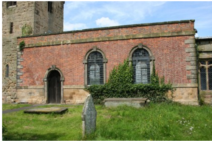
Flemish bond brickwork at St. Andrew's Church c1739
