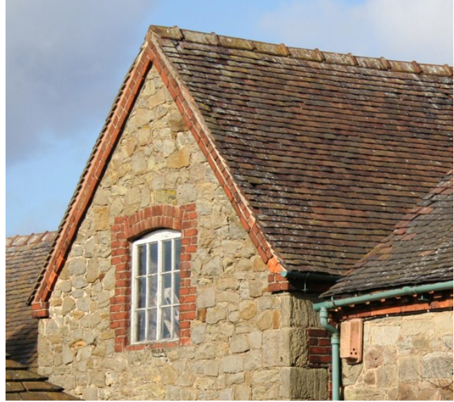
Above - plain corbelled brick verge, eaves and brick quoined window surround, in combination with rubble gritstone walls, at Pool Farm.
