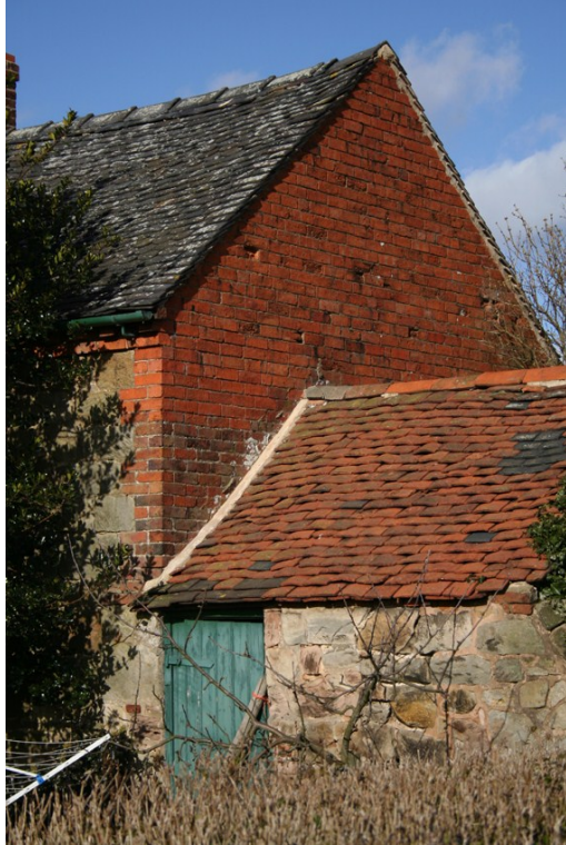
Above - plain close verge and mortared flaunching at Pool Farm.
