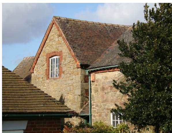
Pool Farm - mellow tones of local stone, finished in brickwork to form straight eaves and verges
