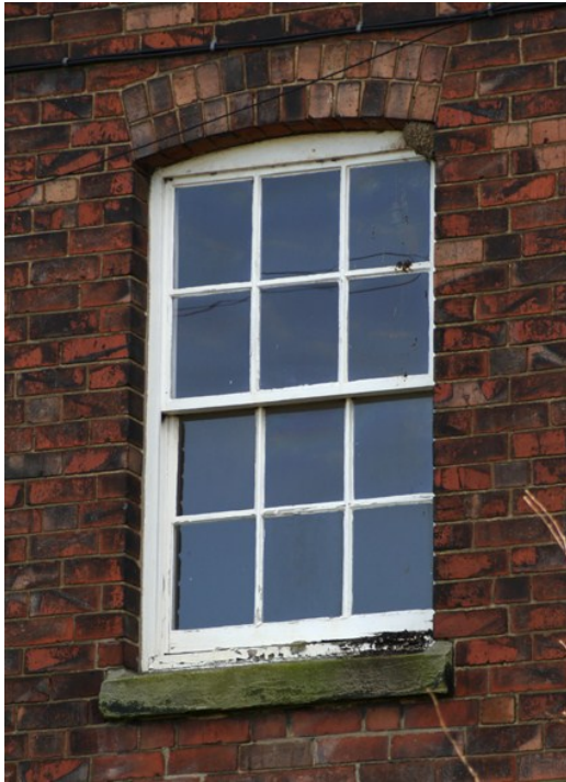
Above - small-paned vertically sliding sash window of 1884 (Woodhouse Farm). During the latter part of the C19 a number of properties were updated with multi-paned sash windows.
