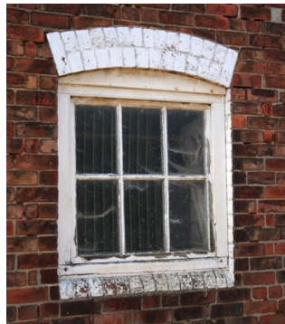
Below left - side-hinged, multi-paned timber casements at Woodhouse Farm Cottage, recessed lights within a chamfered frame. Below centre and right - casements at The Malthouse and Common Farm Cottage.
