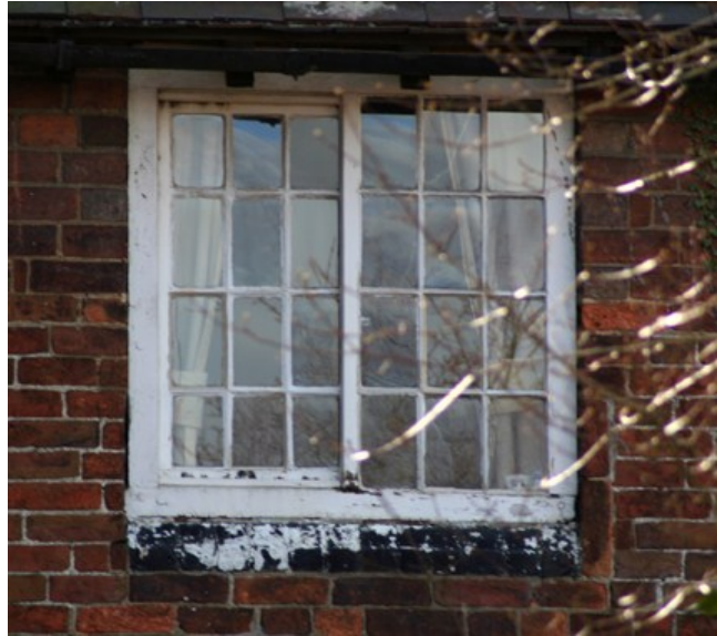
Above - multi-paned horizontally sliding sash window. This pattern is sometimes found on the Melbourne estate properties in the area, but is uncommon (Tutholme).
