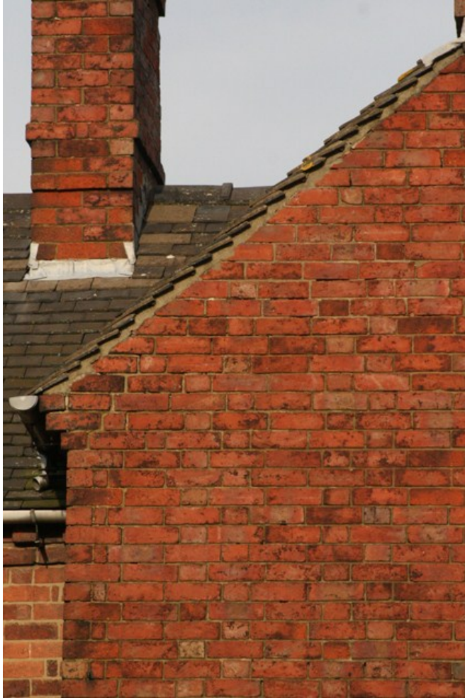
Below - gable-fronted elevation of the former chapel on Chapel Lane. The corbelled and dentilled brick verge continues part way along the front elevation.
