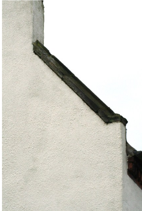
The majority of roofs within Smisby are steeply pitched and finished with a plain close verge, where the tiles simply overlap the brickwork or render (see example on the left).
