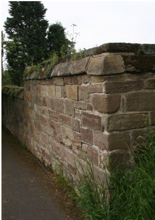
Below left - coursed sandstone boundary to Smisby Manor, with chamfered double-course stone coping. Below right and bottom - rubble sandstone walls, one mortared, the other laid semi-dry.
