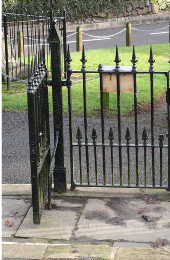
Above left and top right - cast iron railings and gates with spear-headed finials at St. James Church. Above right - hooped steel railings with finials at Hamilton House, Chapel Lane.
