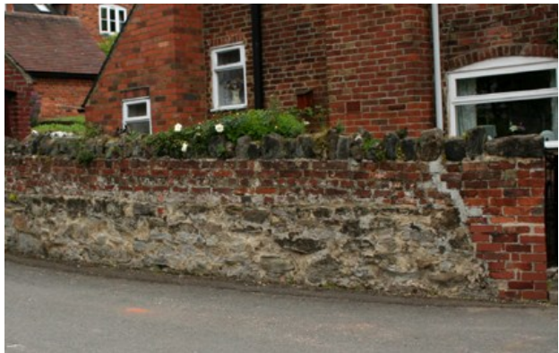
Below left - coursed sandstone boundary to Smisby Manor, with chamfered double-course stone coping. Below right and bottom - rubble sandstone walls, one mortared, the other laid semi-dry.
