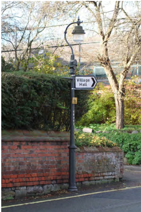
Above - Cast iron lighting columns
