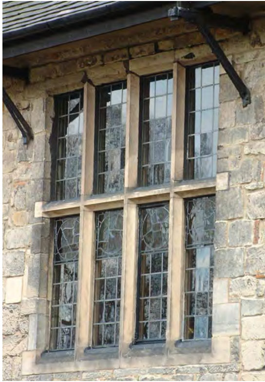
Above - The Old Priory - mullioned windows with stained and painted glass. The leaded lights are fixed directly into the stonework and held in place with "saddle bars".
