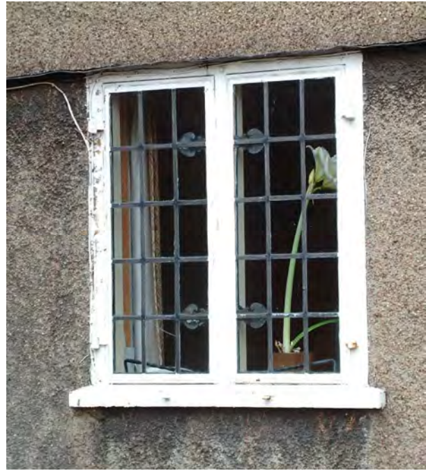
The first windows were made with glass "quarries" (square or diamond-shaped pieces of glass), separated by lead "comes". The lozenge shape evolved as a result of the process of making crown glass. By the 18 th century, glass quarries were usually rectangular in shape (as at The Old Priory - left).
