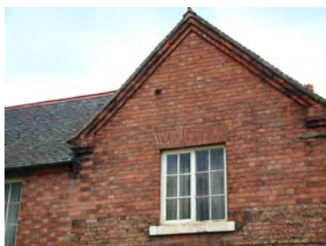
Left - pitched roof with corbelled brick verge
