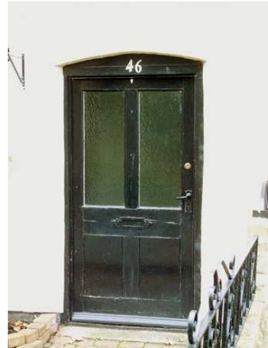
Four-panel door with simple “bead” mouldings (right).
