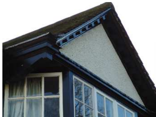
Timber gable (right) with timber dentil moulding, timber console bracket and roughcast render. After about 1910, roughcast render became fashionable throughout the country, largely influenced by the architecture of Charles Voysey and the Arts & Crafts movement.
