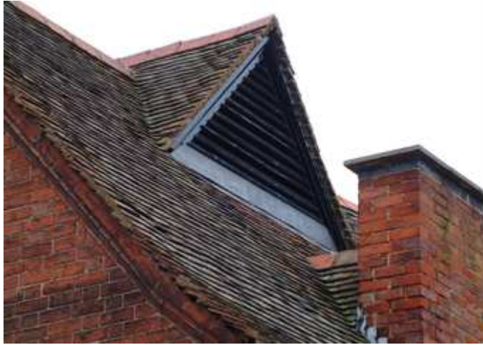
Left - timber ventilator at the old school. This distinctive feature of the late 19th century is combined in the red clay tiled roof with swept valleys.
