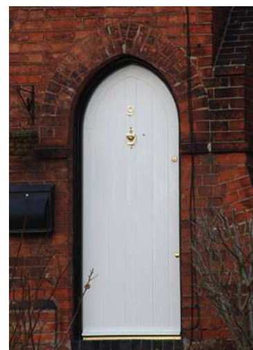
The Gothic Revival introduced a range of doors - nine-panel within a pointed arch (left), plank door with applied fillets and pointed Gothic arches (above centre) and boarded within a pointed arch (above right).
