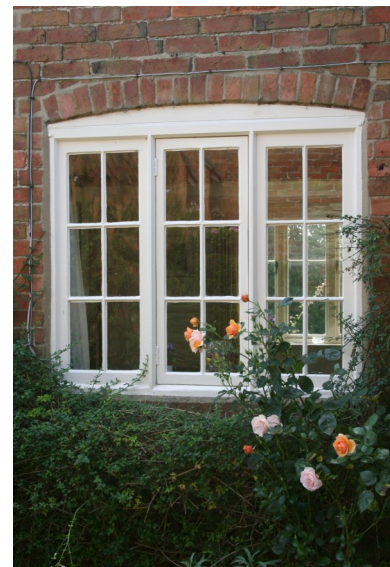
Early 19th century casement "estate" window with chamfered frame at Lane End Cottage
