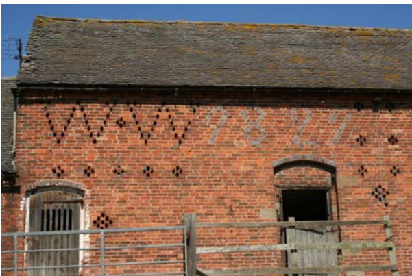
Initials “W W” for William Woodward incorporated as a ventilation pattern and blue bricks laid in a pattern that marks out 1821 at Ivy Close Farm
