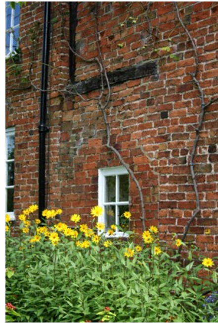
Tatlow's Cottage - the remains of a former bread oven and the timber frame are still evident
