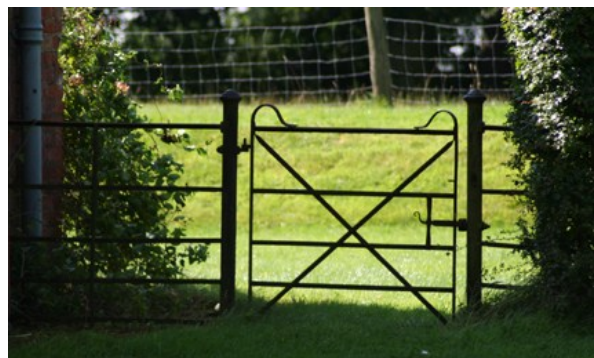
Below - wrought iron five-bar gate and railings with cast iron posts separates the Old Hall from the Village Hall.
