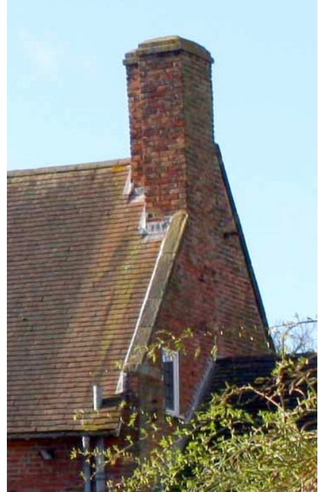
Above - raised coped gable with stone coping at the Old Hall.
