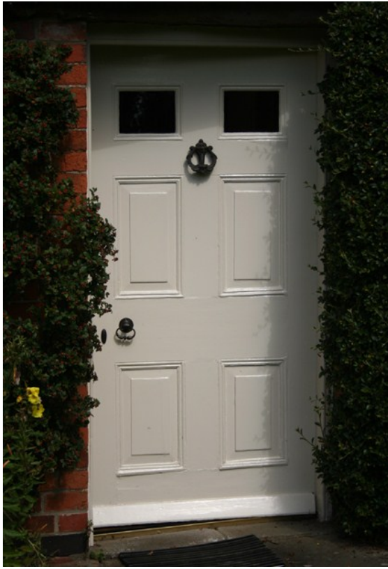
Above - 6-panel Georgian door at Lane End Cottage, incorporating raised and fielded panels and applied mouldings.
