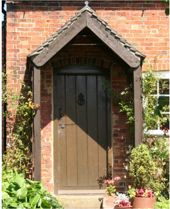
Above - vertically boarded door at Eaton's Cottage, a common style for small estate cottages.
