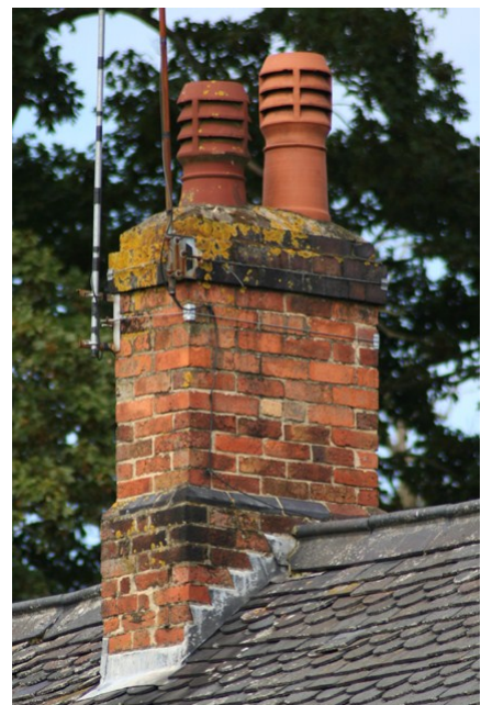
Right - the chimney stack at Eaton's Cottage is more unusual and incorporates brindled brick oversailing courses and a chamfered blue brick weathering.
