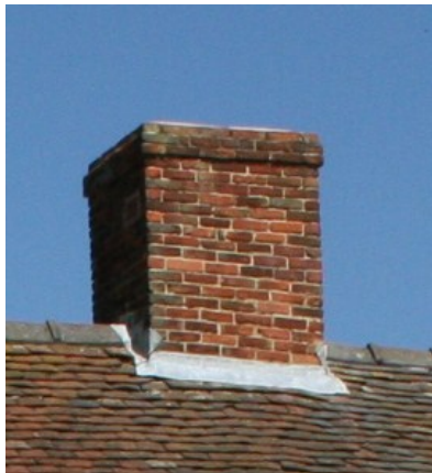
Right - the chimney stack at Eaton's Cottage is more unusual and incorporates brindled brick oversailing courses and a chamfered blue brick weathering.
