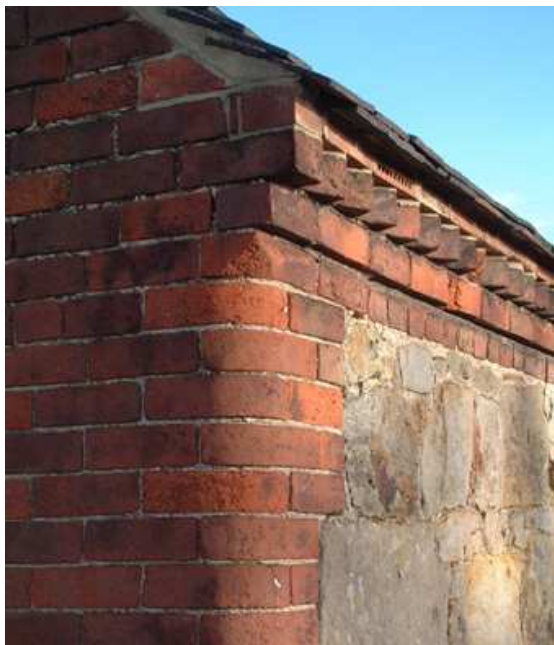
Rounded moulded bricks - used in conjunction with brick chimney stack (right) and corner of agricultural building (above)
