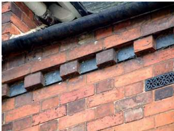
Above and right - the pattern of ventilation holes within brickwork is distinctive. They are survivals from the original use of buildings as hay barns. Most of these slots have been blocked up with slate or blue bricks when the buildings were converted from agricultural uses into dwellings.
