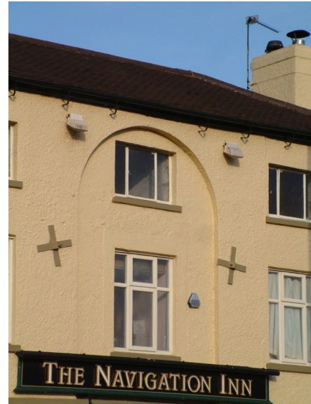
Loss of sash windows and textured render
