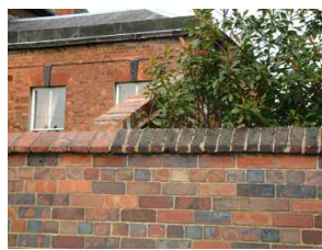
Half-round and triangular coping details (above).
