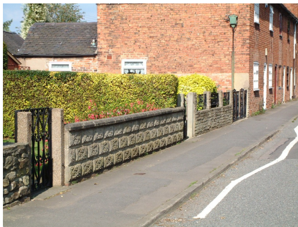
Loss of original boundary walls and replacement in concrete
