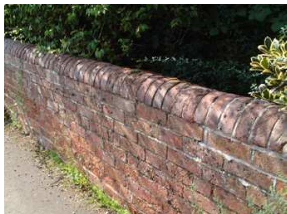
Red brick walls with triangular coping (left) and stone coping (below).
