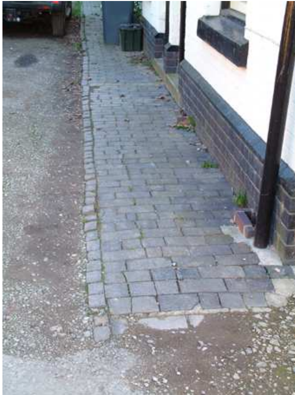
Limestone setts in squared blocks form an apron to the Dog and Duck (above).
