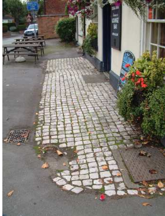
Limestone setts in squared blocks form an apron to the Dog and Duck (above).
