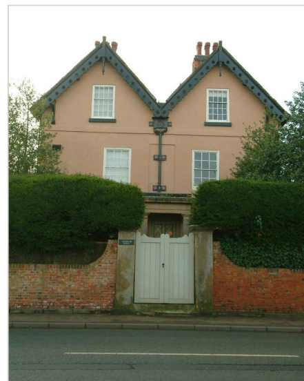
Shardlow House, London Road
