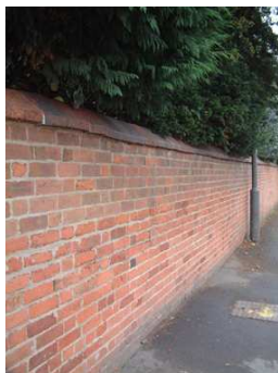
Half-round and triangular coping details (above).
