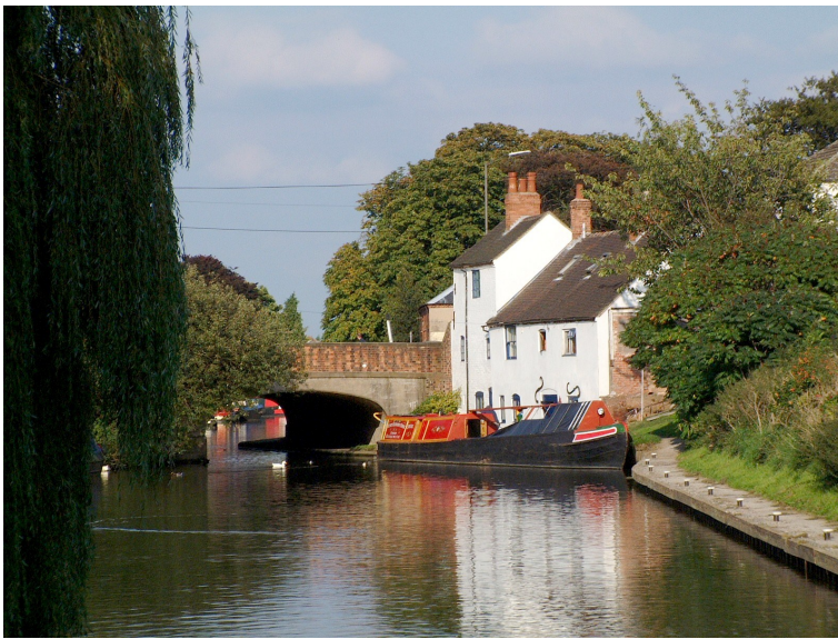
View of Canal Bank and Canal Bridge from Shardlow Lock
