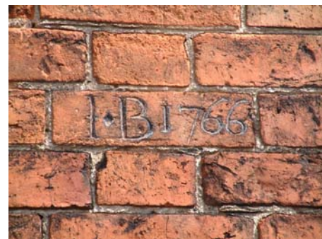
Initialled and dated brick at Brook Farm, built by the Brown family in 1766
