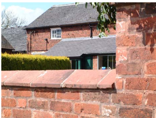
Boundary wall at Common Farm
