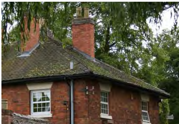
Above - another old roof type is the raised coped brick gable, also found at Lullington Hall.
