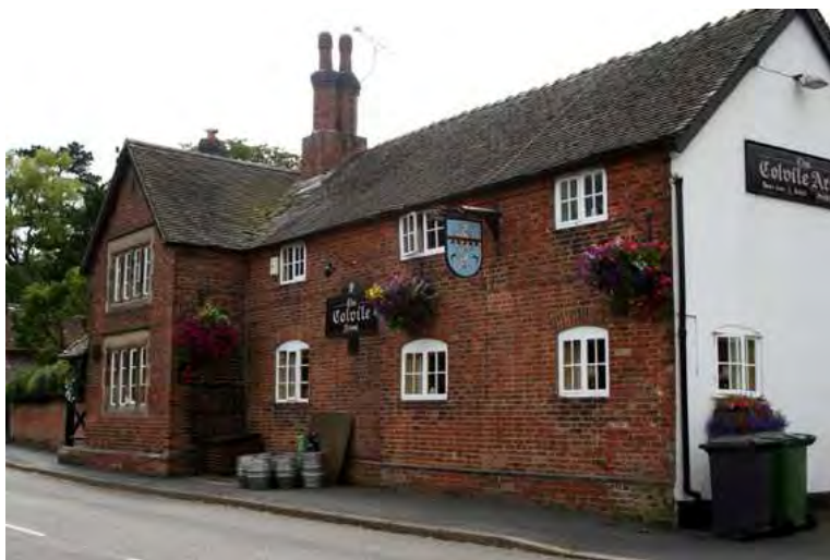
The Colvile Arms 18th century brickwork incorporating dentilled eaves
