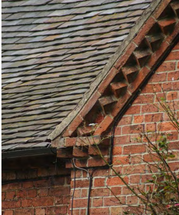
Above - sawtooth and corbelled brick eaves and verge creates a dramatic, detailed profile at Rose Cottage.
