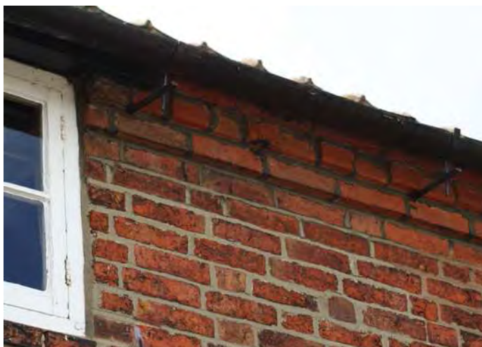
Left - Colvile Arms; dentilled brick eaves. There are several types of decorative brick eaves within the village. Some of the earliest used brick corbelled out in a “dentilled” or “sawtooth” pattern.
