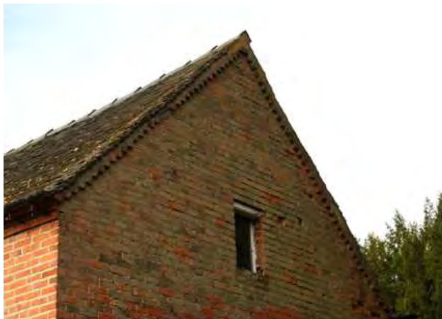
Above - sawtooth and corbelled brick eaves and verge creates a dramatic, detailed profile at Rose Cottage.
