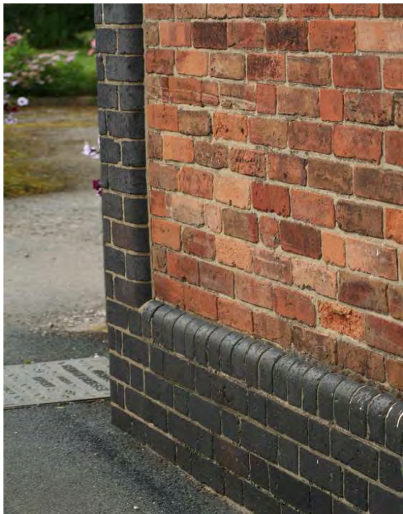
Below left - horseshoe and buttress in blue bricks at the former forge and below right - moulded blue bricks were used for the plinth and pier at The Creamery.
