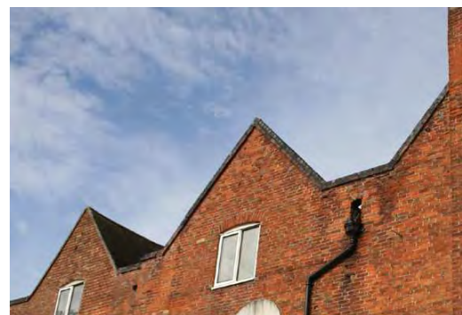
Above - another old roof type is the raised coped brick gable, also found at Lullington Hall.
