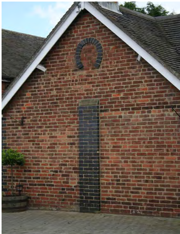
Below left - horseshoe and buttress in blue bricks at the former forge and below right - moulded blue bricks were used for the plinth and pier at The Creamery.
