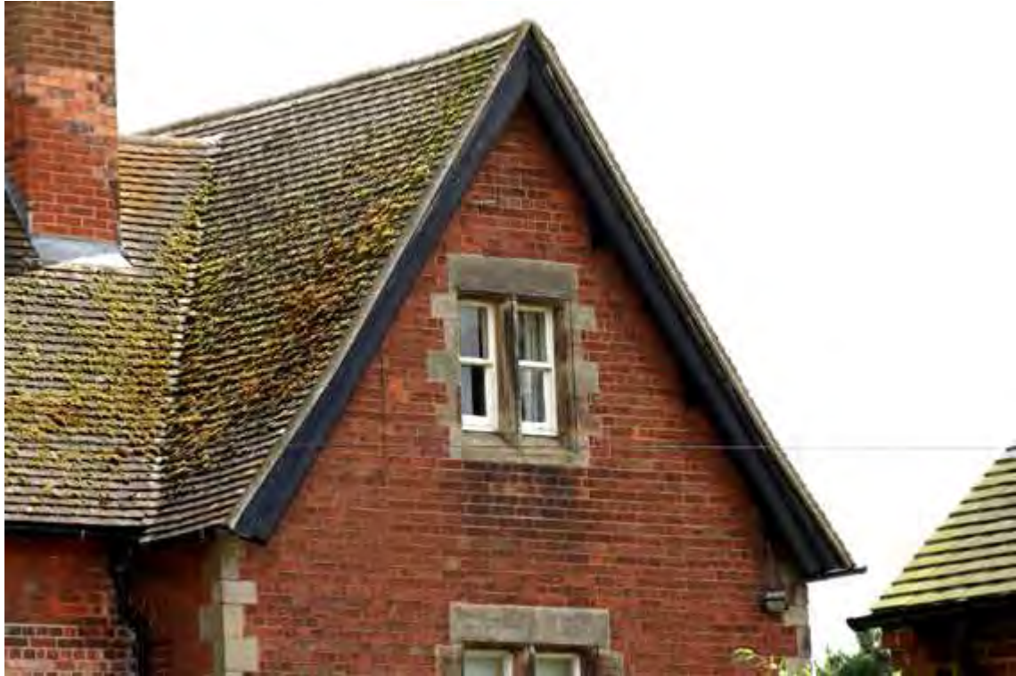
Above - steep pitched roof with timber bargeboards at The Old Rectory (1863).
