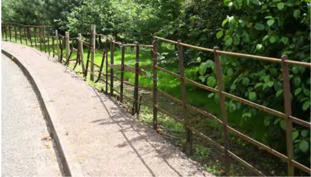
Above - estate railings of wrought iron with round bar top rail and flat bar lower rails (Church St). This type of five-bar estate railing is found in a number of places, but mainly between the private grounds and fields around the former Netherseal Hall
