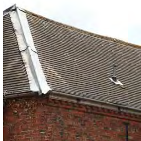
Bottom left and right - hipped tiled roofs at Netherseal Old Hall and The Stable Yard. These hips have rolled lead flashings.
