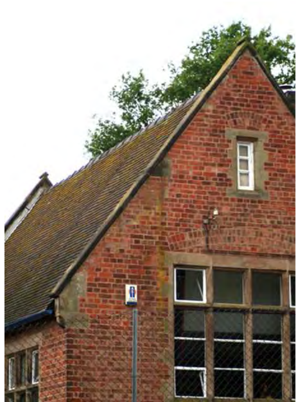
Left and bottom left - stepped and raised brick parapet gables (The Old Hall and The Old Stableyard).
