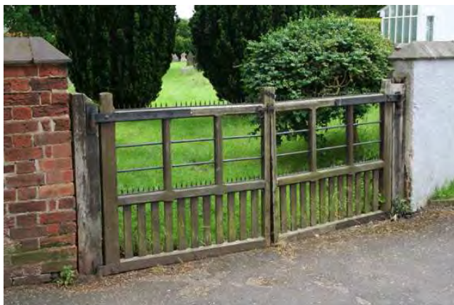
Left - timber gates with chamfered mouldings and spiked wrought iron rails to the new churchyard on Main Street
