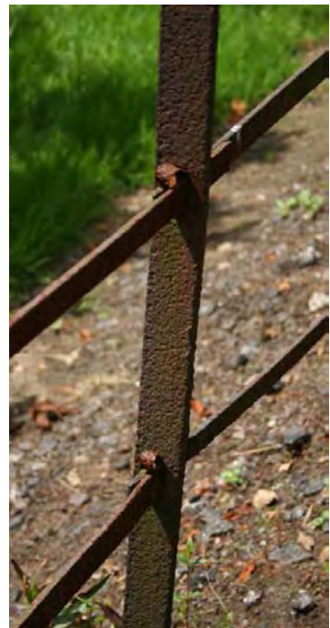
Left - early C20 wrought iron railings fixed to brick wall at the Village Hall, Main Street
