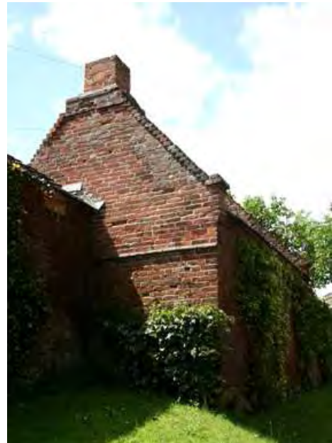
Stepped brick parapet to roof at Grade II listed former Smithy at the Old Stableyard
