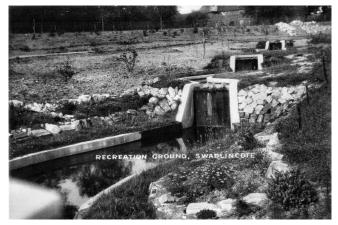
The cascade was designed as an ornamental water feature, lined with concrete and a number of stone ledges to provide a series of small waterfalls. Rockery style planting along the margins soften the banks. This was laid out and completed in July 1934. The water from the cascade fed the paddling pool – a large diamond shape as seen in the photograph (the original kerb edging of the paddling pool can still be found). This was a very popular feature on hot, sunny summer days.
