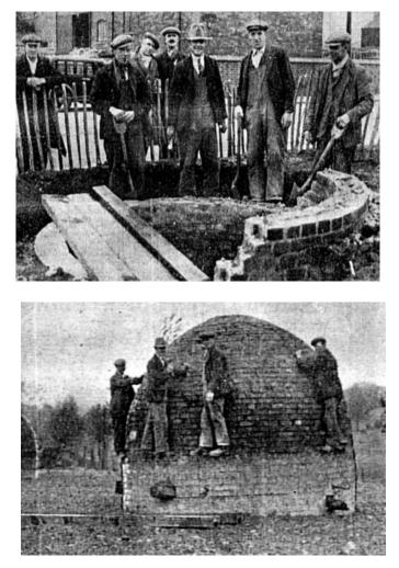
The mine was served by a mineral line from the main railway that ran through Swadlincote, south of the present park. Remains of an old railway bridge can be seen on the access path from Belmont Street. The mine shafts were capped off as shown in the photographs above from Burton Mail dated 6<sup>th</sup> June 1938.
