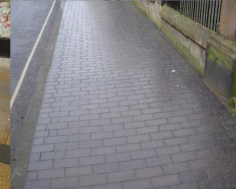
▲ Staffordshire Blue clay brick paving and stone kerbs used in town centre improvement scheme
