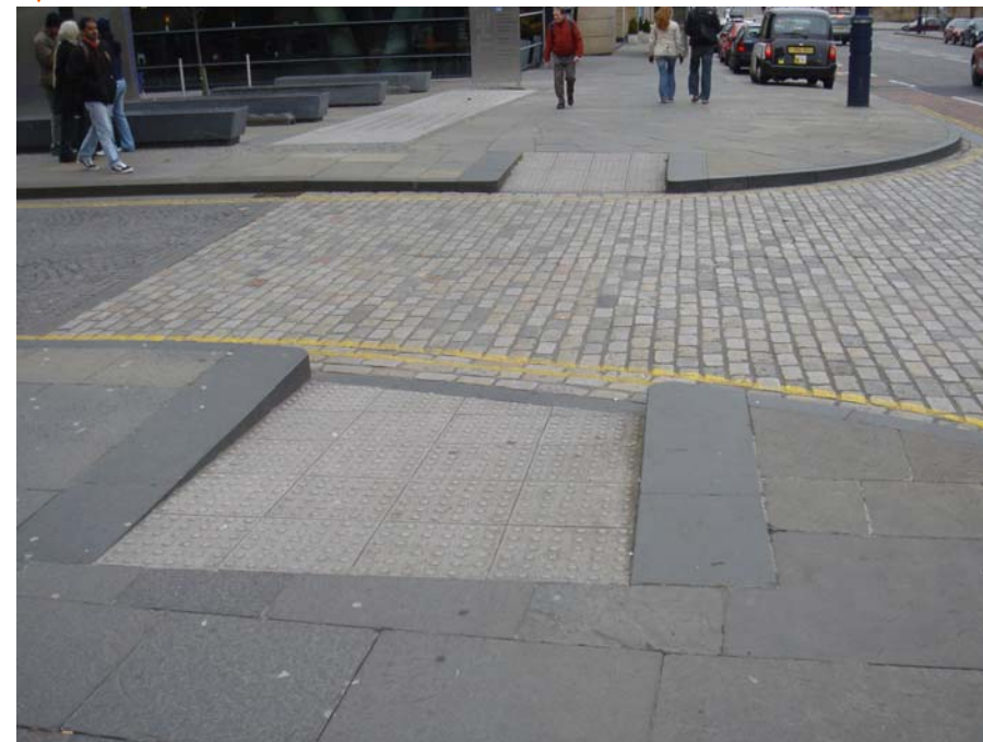
▼ Dropped kerbing and tactile paving - Edinburgh
