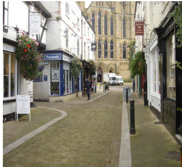
▲ Footpaths and road reinstated using yorkstone split and cropped setts with low rise wide profile granite kerb and dished sett drainage channel
