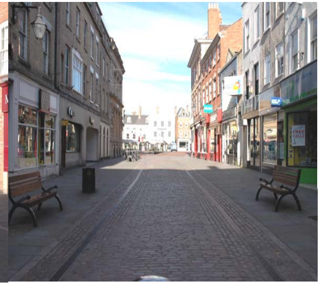
▲ Recent street refurbishment using yorkstone flag paving for footpaths, granite setts for roadway, with flush granite kerb edge and wide sett drainage channel with linear cast iron drain cover
