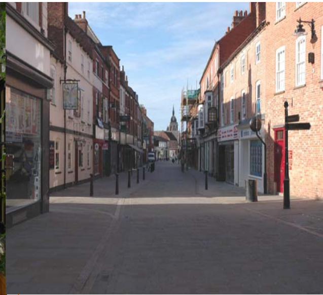
▲ Recent town centre refurbishment using yorkstone flag paving for footpaths, yorkstone setts for roadway, with low rise granite kerb edge and drainage channel
