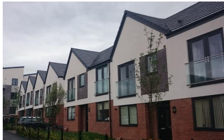
Contemporary architecture with traditional scale and massing replicating nearby terraces and sawtooth roofline of nearby industrial units: Rose Hill, Woodville, Swadlincote
