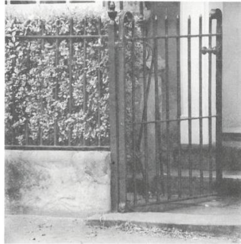
Traditional cast iron railings and gate.
