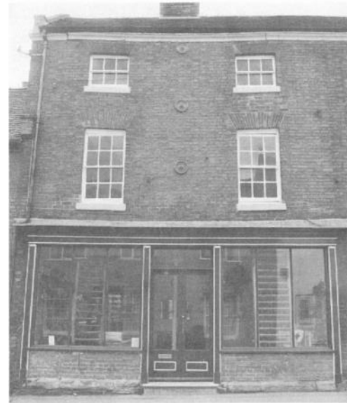
Rebuilding the front of this Grade II Listed Building has been avoided by using steel supports and straps which are largely concealed
