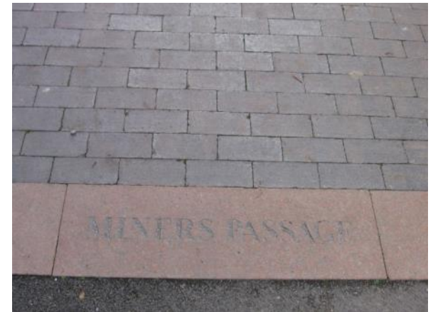
Staffordshire blue clay bricks and granite threshold strip with historic reference: Swadlincote town centre
