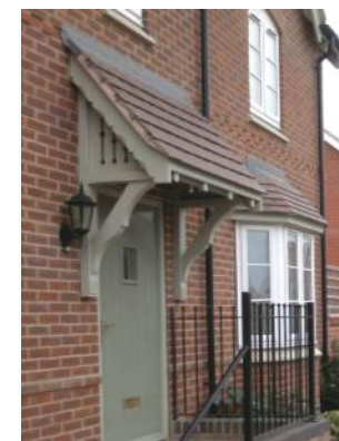
Castleton Park, Church Gresley: Timber door canopy
