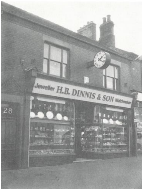
Early 20th century shop front with curved glass and cast iron mullions in Swadlincote.
