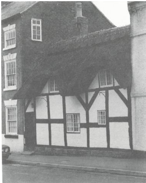
Potter Street, Melbourne. 16th century timber frame.
