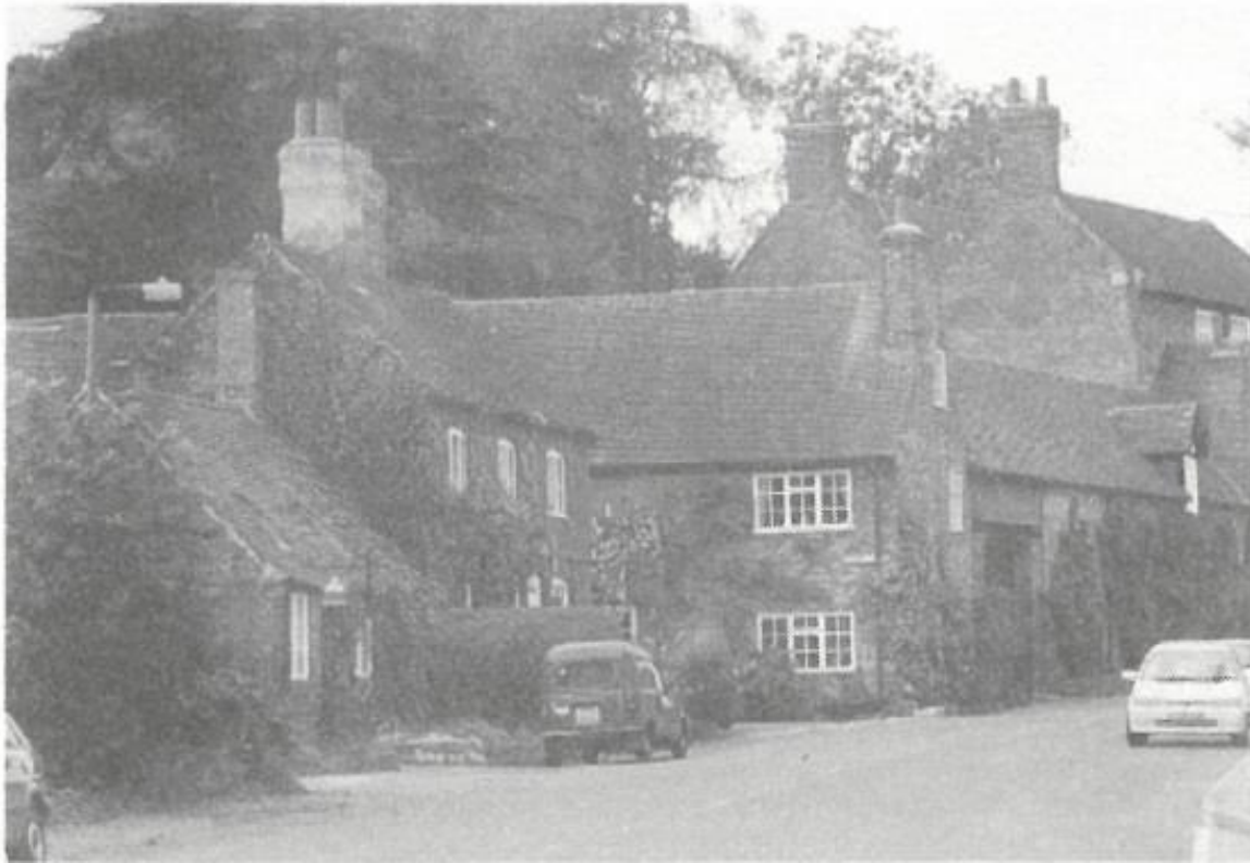
A typical grouping of traditional buildings in Melbourne. The building in the centre of the picture has unfortunately lost its original window
