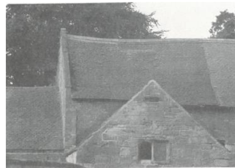
Melbourne Tythe Barn. A mixture of brick, stone, machine made and hand made plain clay tiles.
