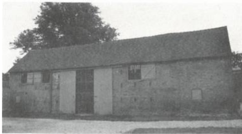
Former threshing barn, now a restaurant at Calke Abbey. Notice the 'breathers' on either side of the large doorway.
