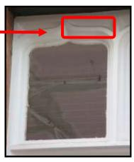
**The Spandrel** is the space between two arches or the space between an arch and a rectangular enclosure
