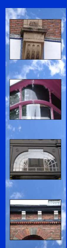
racket A structural piece of stone, wood or metal jutting from a wall which carries the weight of the material above.
