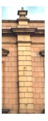
uoins Blocks of brick, stone or concrete featured on the corner of a building. In some cases they strengthen the wall. Sometimes they can be used decoratively to make a feature of the corner of the building.
