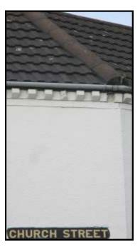
aves: the lower edges of a roof at the junction between the roof and walls. They can be designed to jut out so that rain water is thrown clear of the building and does not run down the walls. They are often decorative as well as functional.
