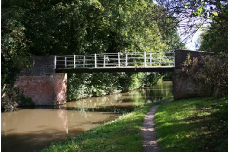
Above left and right - pedestrian footbridges over the canal. Bridge No. 10 at Cliff Wood (left) was always a narrow footbridge, which also catered for packhorse traffic approaching the river crossing. The iron posts and rails are 20th century and may have replaced a timber fence. The footbridge at Weston Lock (right) has a cast metal deck and is a pattern repeated at the locks.
