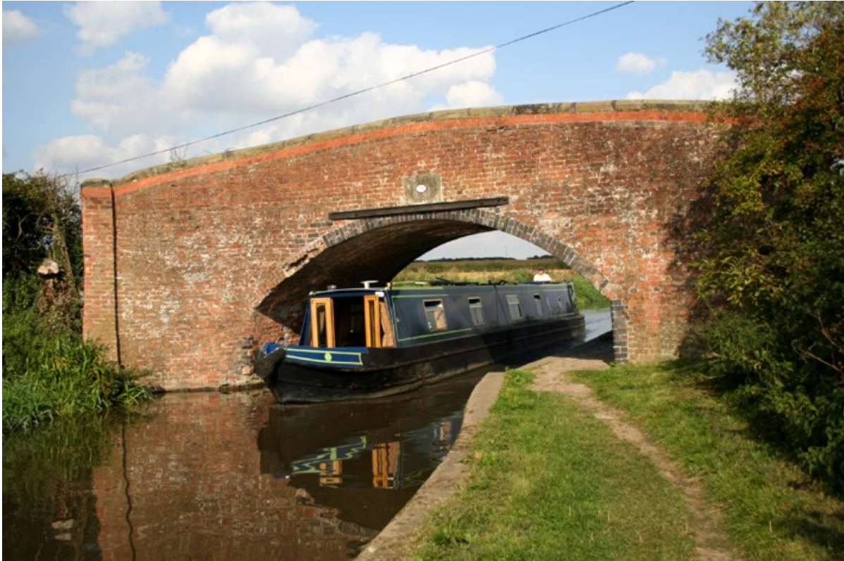
A typical canal bridge. Stone coping to red brick structure. Later repairs in red and blue engineering bricks.
