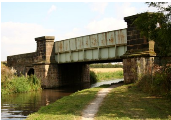
Below - railway bridges over the canal. Left; bridge near Stenson Junction incorporates giant stone piers with rusticated stone bases and cornices and riveted iron plate box-girder construction. Right; smaller scale bridge of similar construction at Weston Lock, with handrail to parapet.
