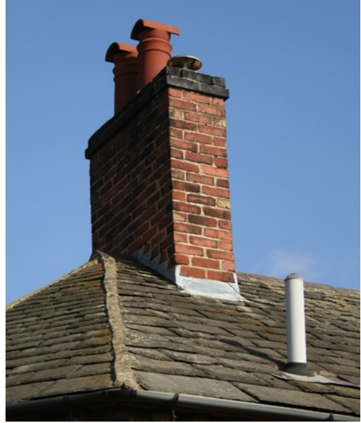
Left - brick stack with rounded moulded corners (Stenson Lock - Harpur Crewe estate). Blue brick oversailing courses (above) at Swarkestone Stop.
