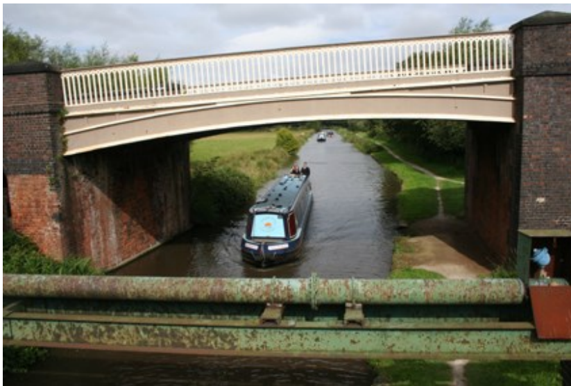
Below - railway bridges over the canal. Left; bridge near Stenson Junction incorporates giant stone piers with rusticated stone bases and cornices and riveted iron plate box-girder construction. Right; smaller scale bridge of similar construction at Weston Lock, with handrail to parapet.
