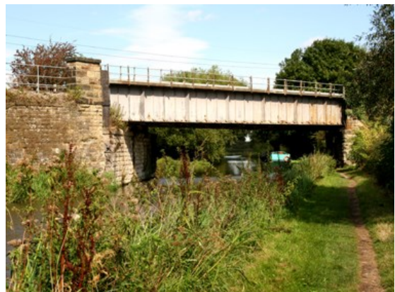
Below - railway bridges over the canal. Left; bridge near Stenson Junction incorporates giant stone piers with rusticated stone bases and cornices and riveted iron plate box-girder construction. Right; smaller scale bridge of similar construction at Weston Lock, with handrail to parapet.
