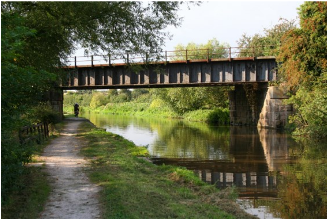
Railway bridge over the canal near Stenson
