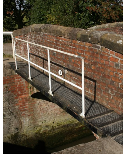
Above left and right - pedestrian footbridges over the canal. Bridge No. 10 at Cliff Wood (left) was always a narrow footbridge, which also catered for packhorse traffic approaching the river crossing. The iron posts and rails are 20th century and may have replaced a timber fence. The footbridge at Weston Lock (right) has a cast metal deck and is a pattern repeated at the locks.
